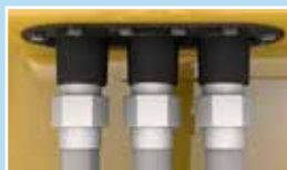
Conduit Threads On Outside of Box*
