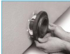
**Step 2:** Insert sections of piping through flexible entry boots and attach to fittings inside the dispenser sump base.
