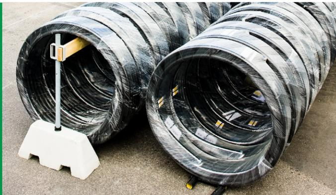
When coils are stored upright they need to be supported to avoid deformation of the pipe.
