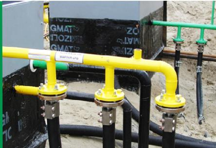
Manifold prepared to be fitted with safety relief valve.
