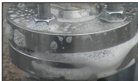
Perform tightness test with soaping before backfill.
