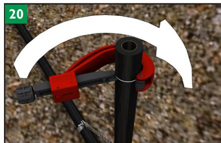
Cut the pipe to its finished length using a KPS rotating pipe cutter.
