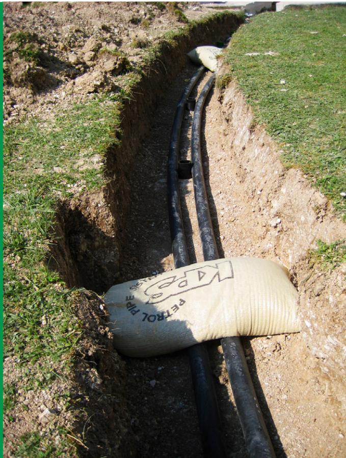
*Use bags with sand to keep the pipes in place during installation.*
