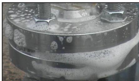
Perform tightness test with soaping before backfill.
