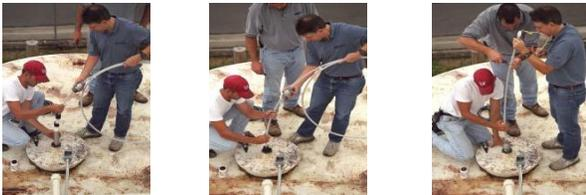
Figure 4-5 Adaptor, Float and Weight Installation
