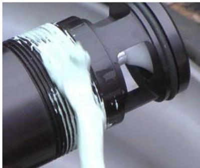
Figure 6-3 Apply Thread Sealant
