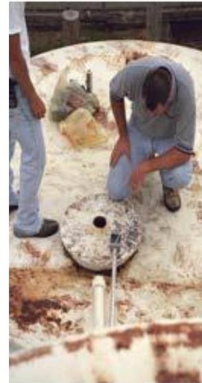
Figure 4-6 Flex Probe Installation
