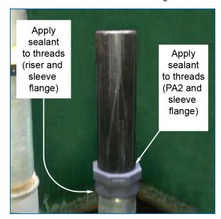
Install the PA 2 inch protective sleeve (purchased option when the XMT-SI-RF is installed in a riser).
