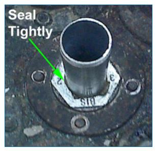
• Seal the threads at the sides of the flange with plumber's hemp and sealant to make a tight seal.
