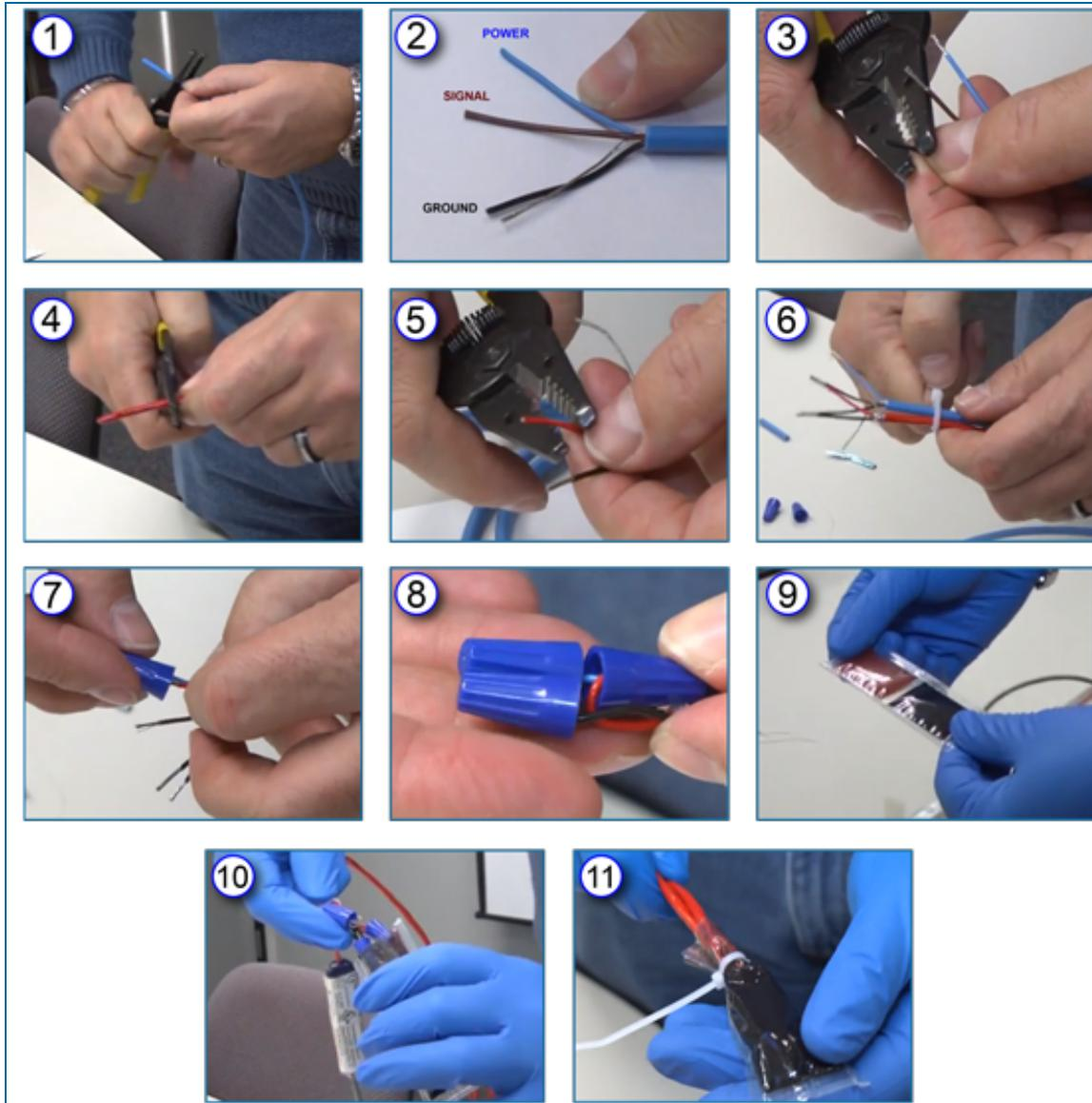
Assembly of the the Epoxy Seal-pack for Waterproof Electrical Connections
