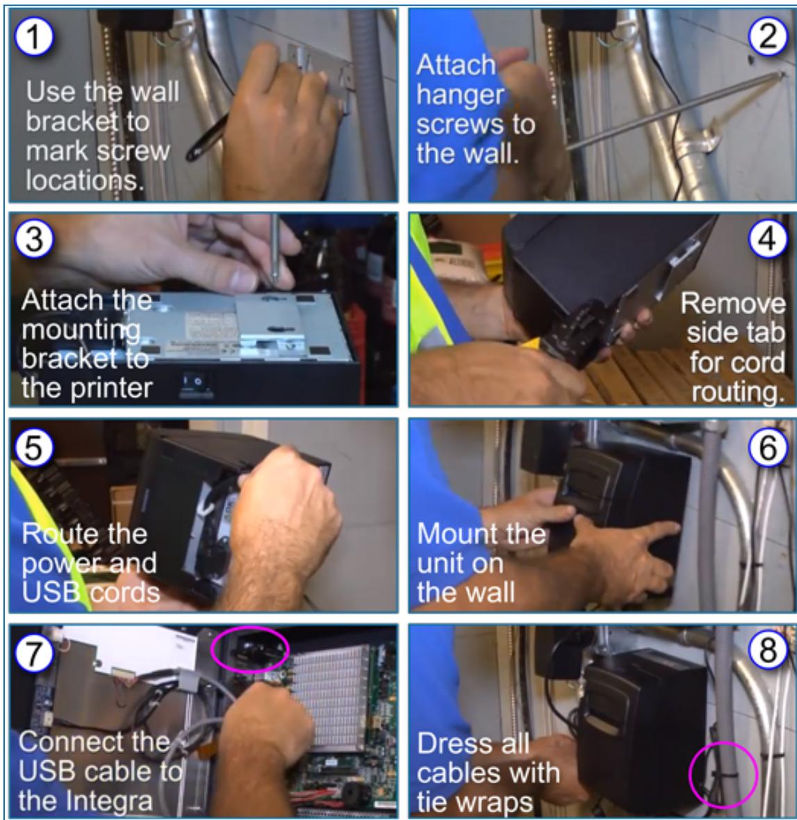
1. Use the Wall Bracket to mark the location for two (2) hanger screws (not included in the kit).
