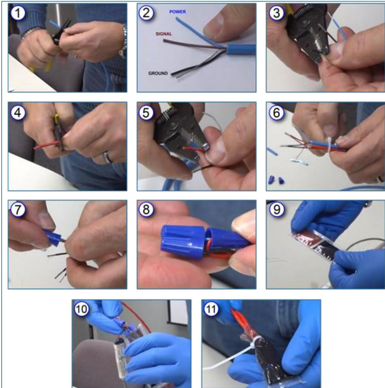
Figure 9-5 Assembling the Epoxy Sealpack for Waterproof Electrical Connections
