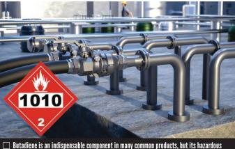
nature means it must be carefully handled at all times. Advanced dry-disconnect technology can aid in that task.
