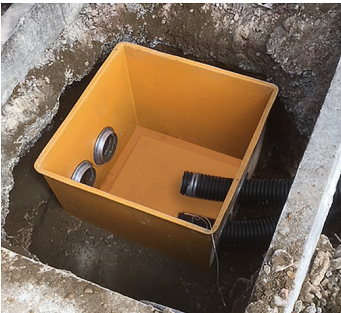
Fibrelite products enable a more efficient site construction
