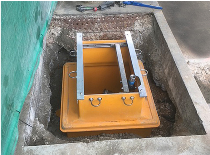
BP required retrofit chamber systems
