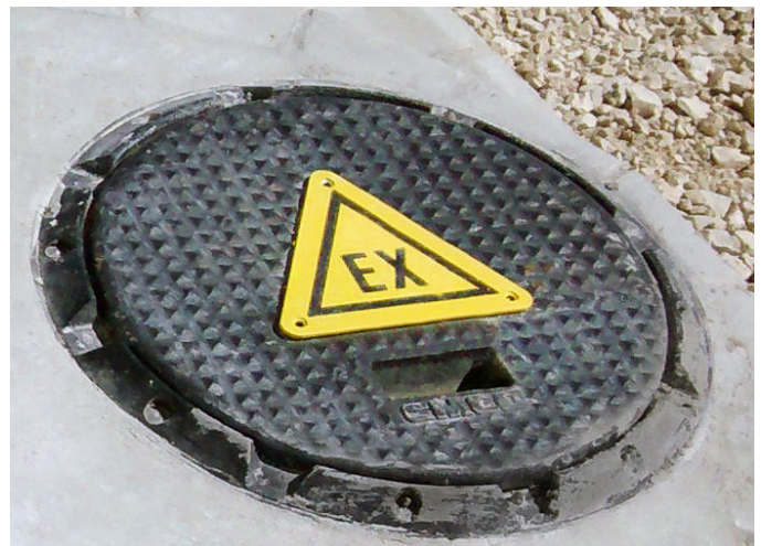
Previously used cast iron spill chamber
