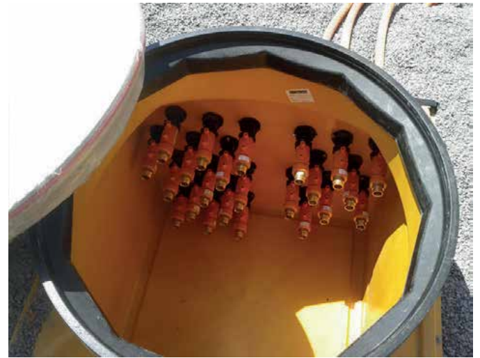
Cable drawpit with 32mm conduit piping
