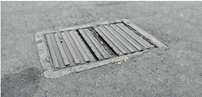
Previously installed steel access pit over water mains valve
