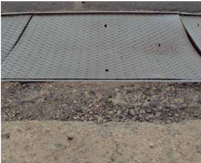
Corroded and deformed: cheap steel covers
