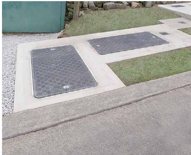
The 25 tonne load tested lightweight covers
