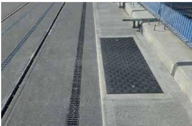
Bespoke trench covers for trackside gear
