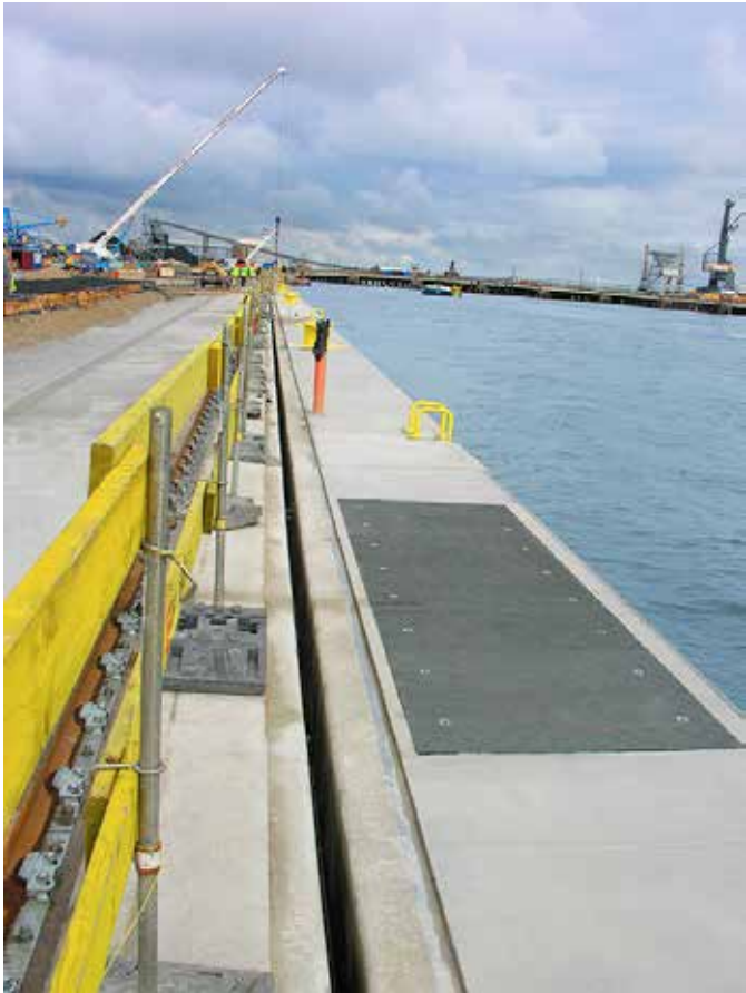
D400 load rated trench covers allowing safe manual removal
