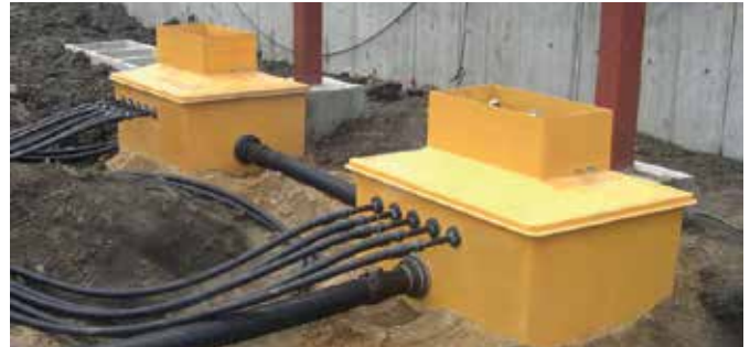
Fibrelite's Tokico AB26L dispenser sumps
