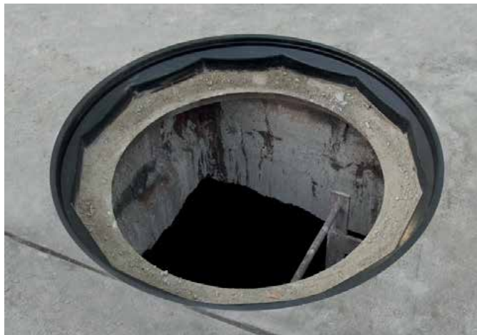
Fibrelite composite frame installed in sidewalk
