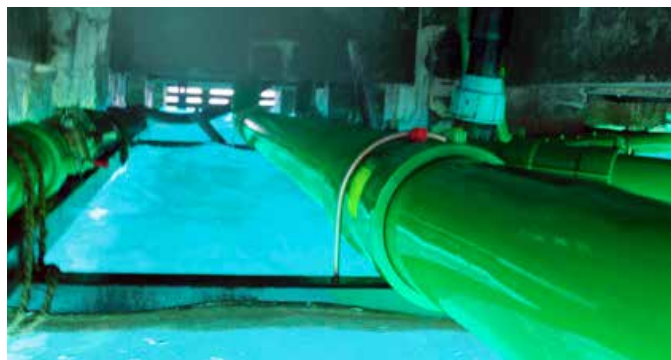
Fuelling lines run below jetty from ship to storage point and are impervious to corrosion from saltwater
