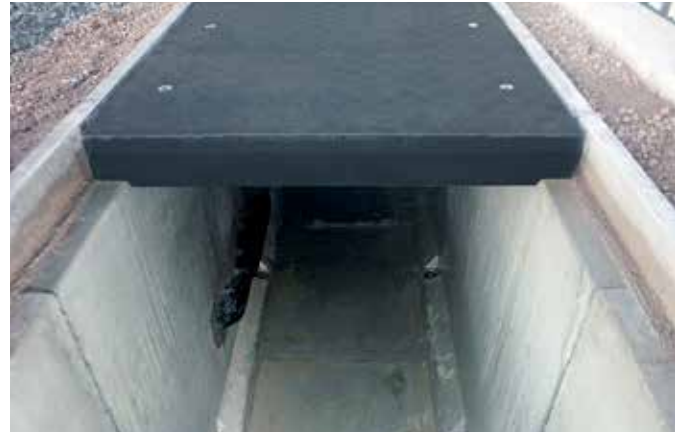
Covers 'stepped' to reduce weight and fit trench width
