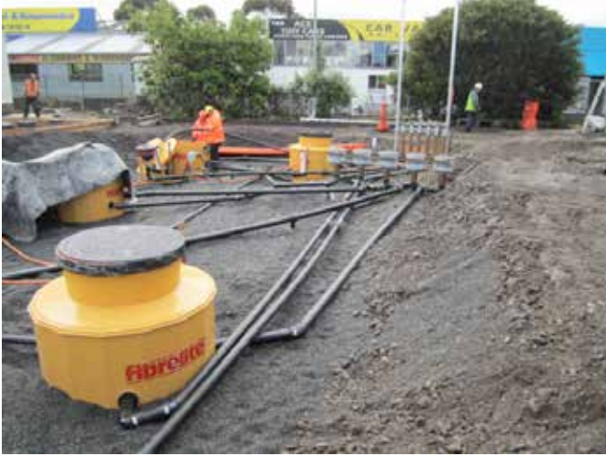
Fibrelite sumps are vacuum testable ensure watertightness
