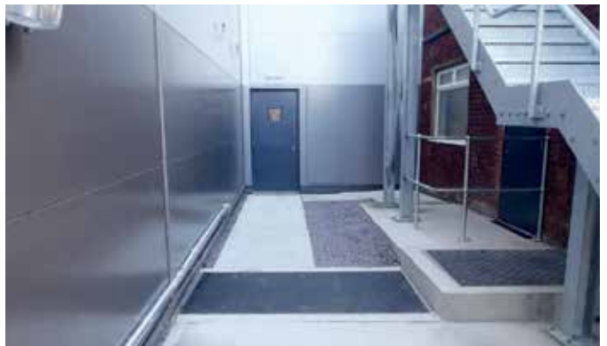
Retrofitted sealed Fibrelite covers installed
