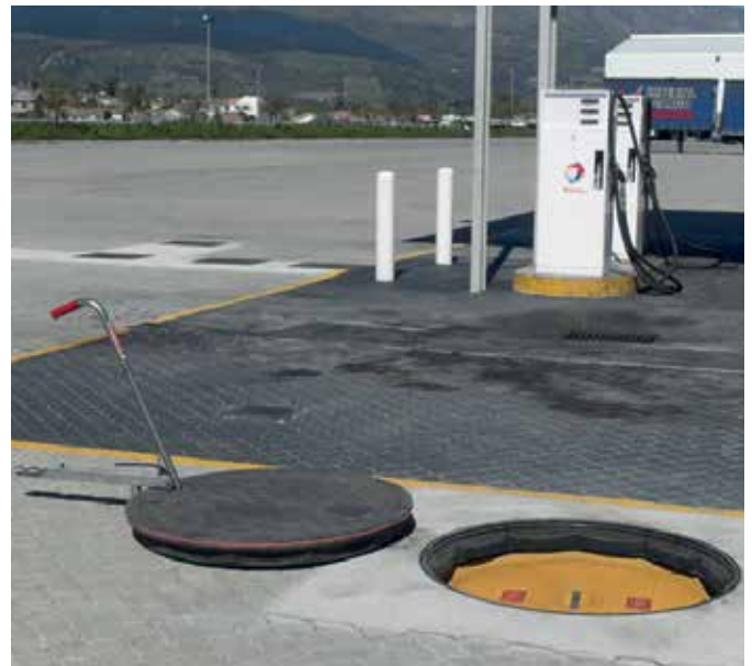
Fibrelite cover with easy to remove FL7A lifting Aid over a 1.2m (42") watertight turbine sump
