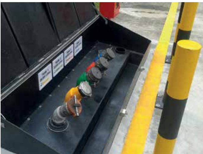
Fibrelite's S22SH-2/AGF above ground remote fill box
