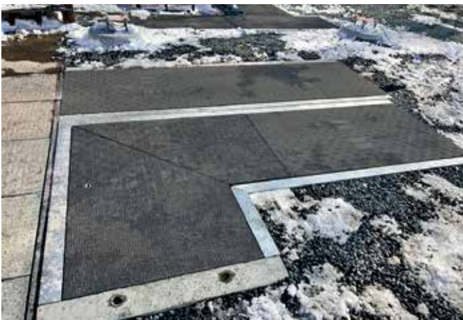
Fibrelite and Trenwa's partnership product offering: light strong access covers inset into heavy duty trenches
