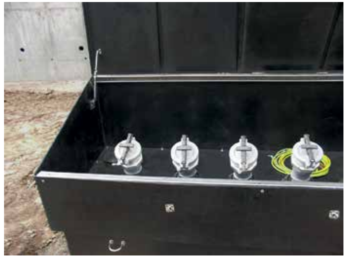
OPW heavy duty corrosion resistant seal caps
