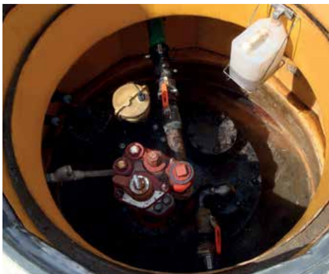
Fibreglass turbine sump with 55" tank collar
