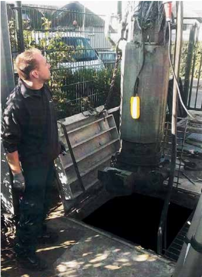
Heavy metal covers requiring 2 men and a crowbar to remove, emanating odours
