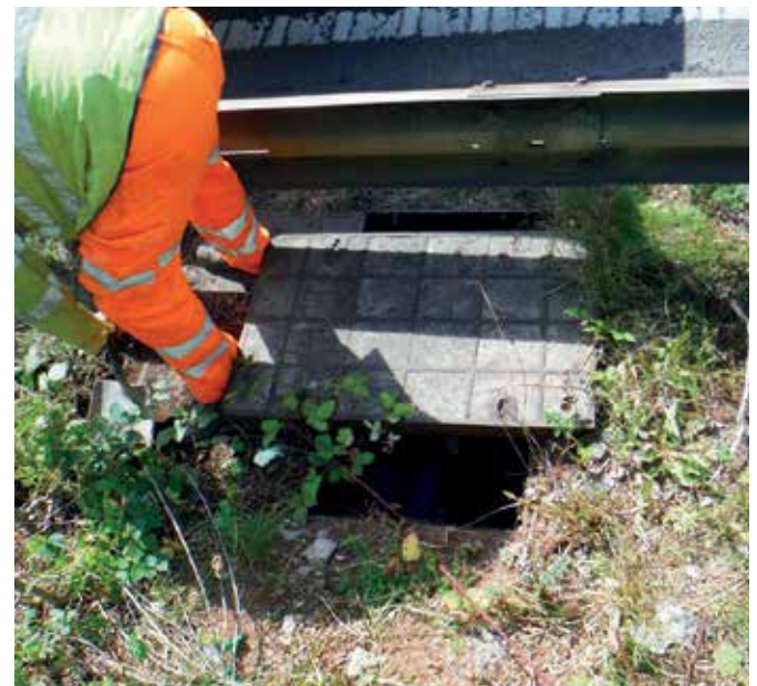
Damaged cast iron and concrete cover
