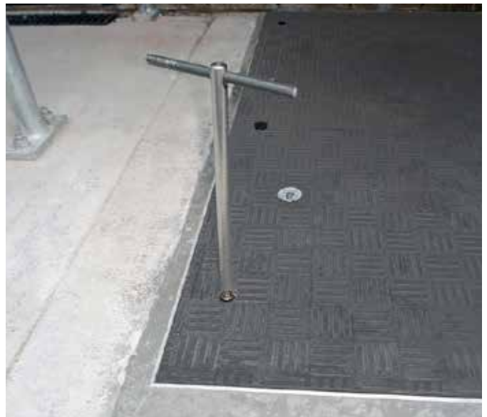
Secured/restrained covers, preventing unauthorised access
