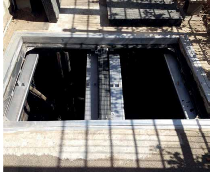
Removable centre beam supports covers
