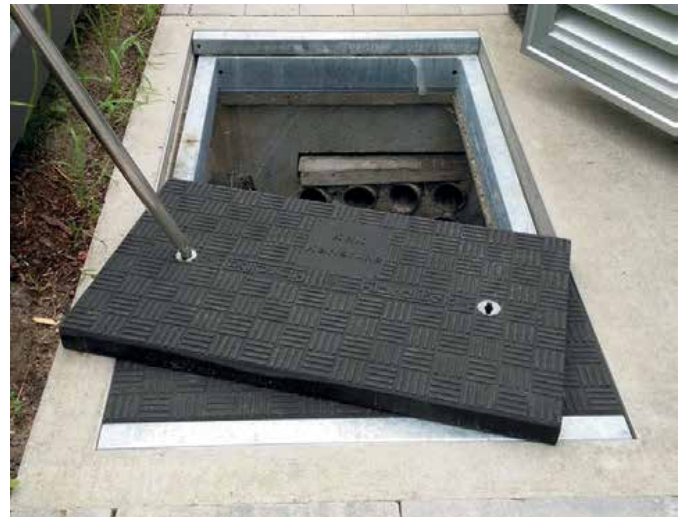
Fibrelite trench panels installed over the chamber
