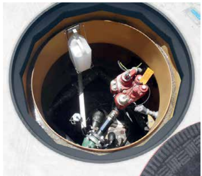
Fibreglass 1.2m (42") turbine sump
