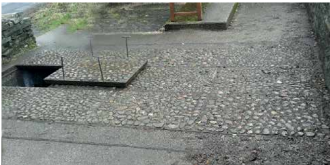
Cobbled covers requiring lifting equipment
