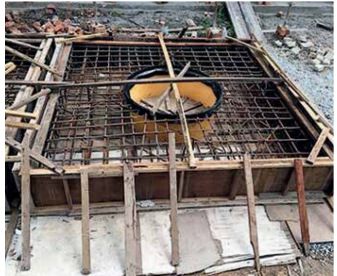
Prefabricating concrete plinth with Fibrelite FL90 frame
