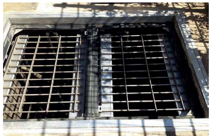
Removable beams hold safety grid
