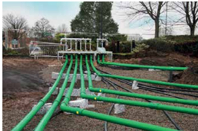
KPS formed bends below fill point
