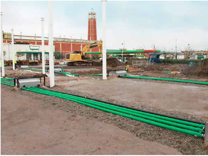
10m lengths of custom 75/63mm KPS straight pipe allowed fast installation without the need for a welding socket in middle
