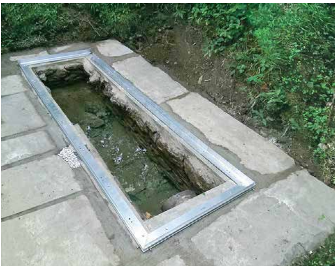
Fibrelite encapsulated frame
