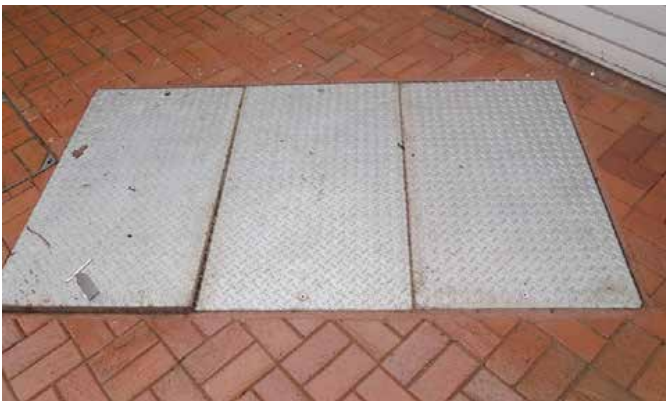
Previously installed odour-emitting galvanised covers
