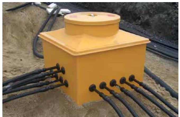
Fibrelite's electrical conduit drawpit being installed
