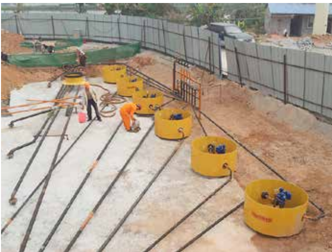
Fibrelite tank sumps (S14-390) being installed
