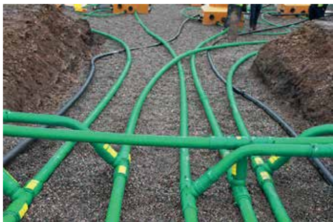
All integrated double wall KPS fittings weld both pipe walls simultaneously
