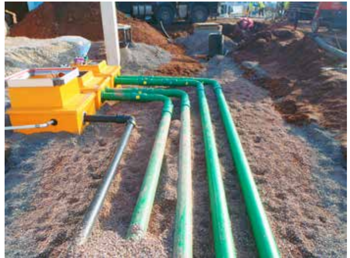
All integrated KPS fittings weld both pipe walls simultaneously
