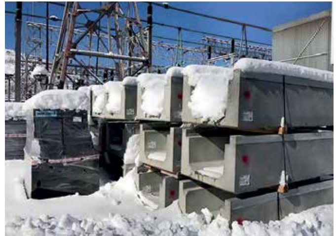
Trenwa's precast trenches ready for installation
