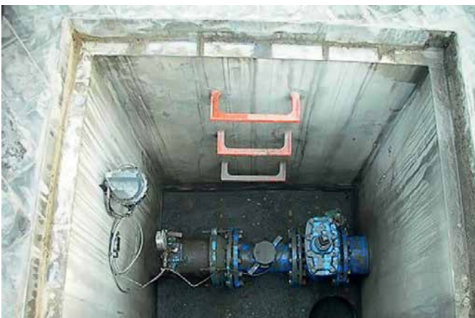
Automatic monitoring system located beneath metal cover which blocked signal. Photo credit: Aguas de Cádiz
