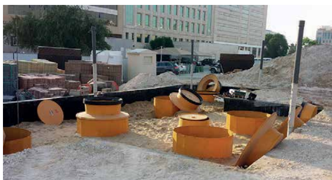
Fibrelite S14-390 tank sumps under installation
