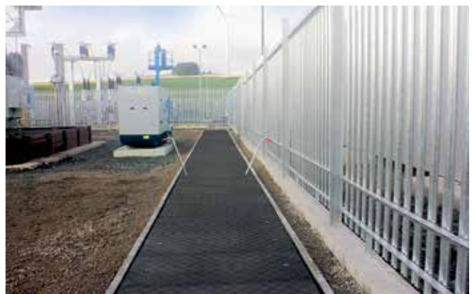
Bespoke Fibrelite trench covers 1250mm span
