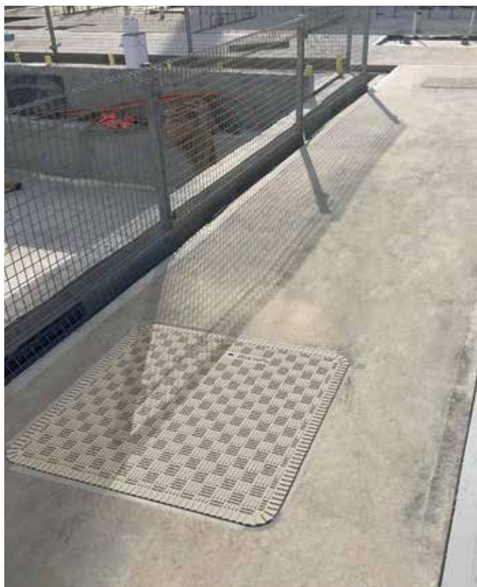
Installed cover over balance tanks
