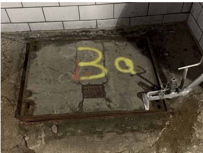
Old unsafe concrete covers
