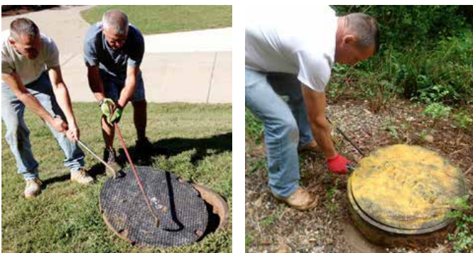
Heavy cast iron covers pose a significant threat of back & shoulder injuries along with the risk of trapped extremities
