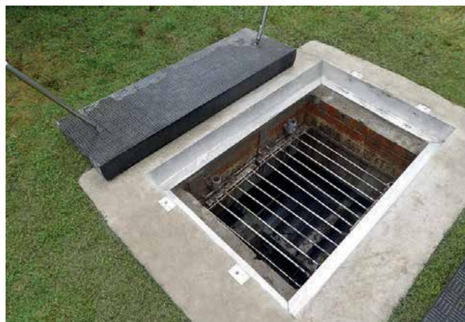
Safe and easy manual removal: Fibrelite FM45 covers are removed by hand from the CSOS (Combined Sewer Overflow System) chamber
