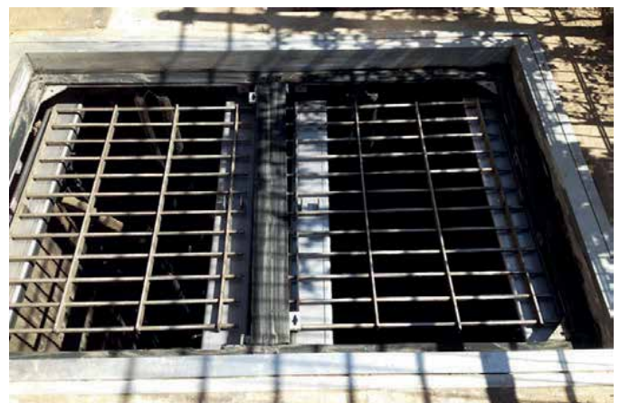
Removable beams hold safety grid
