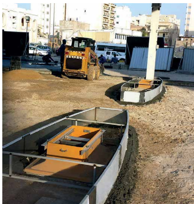
Fibrelite EL-G-E500 dispenser sumps ready for concreting
