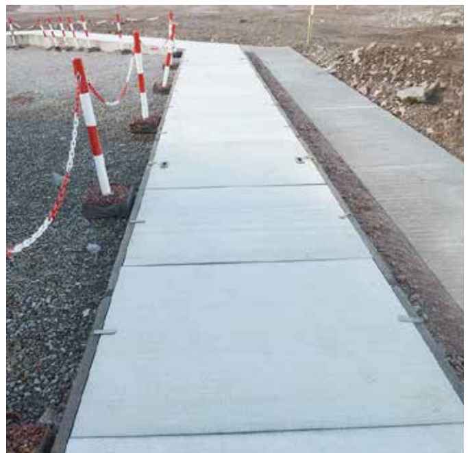
Concrete covers unable to withstand pedestrian traffic
