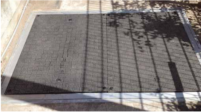
Sealed odour-tight covers installed
