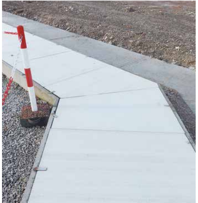
Previously installed low quality concrete covers
