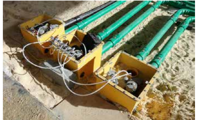
Secondarily contained Fibrelite remote fill sumps
