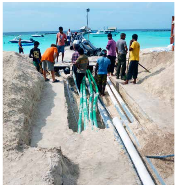
Installer friendly KPS piping allowed for quick easy installation
