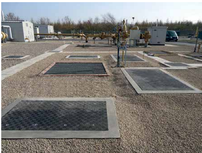
Corroded and damaged cast iron and concrete covers were replaced with Fibrelite's lightweight trench panels
