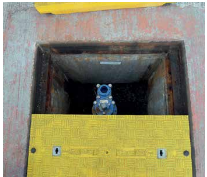
Previously both of the extremely heavy steel covers had to be removed to expose the isolation valve for the drinking water supply. Now only one Fibrelite trench cover needs to be removed.
