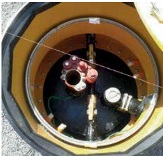
Fibrelite's 1.2m 16 sided turbine sumps being installed
