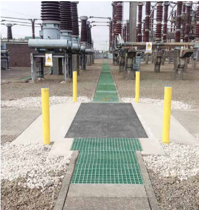
The installed Fibrelite heavy duty trench covers
