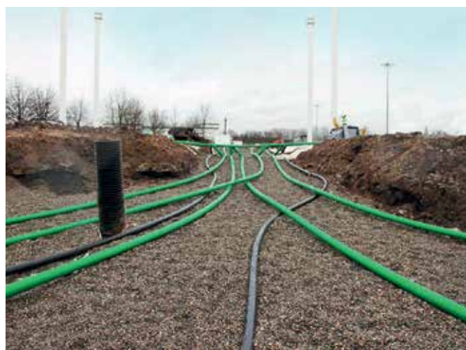
KPS pipe is also available in coils
