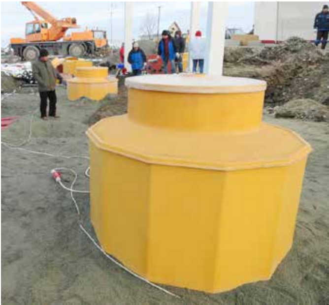
The GRP chambers are fully adjustable to accommodate shallow tank burial depths
