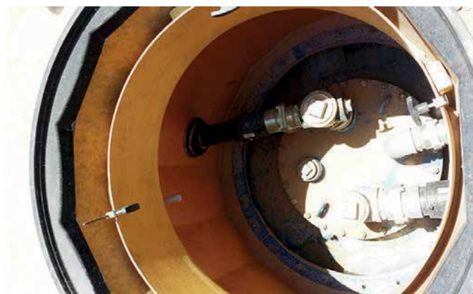
Vacuum testable Fibrelite pipe sealkits form watertight seal
