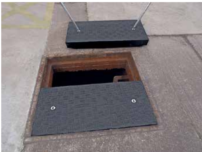
Bespoke Fibrelite covers installed into existing frame
