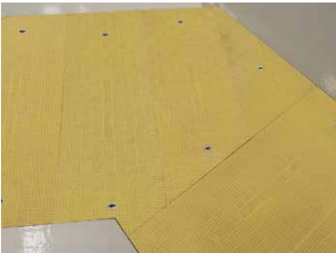
Bespoke trench covers for complex corner sections
