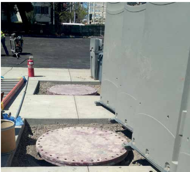
Fire Manway lids (tank buried underneath)
