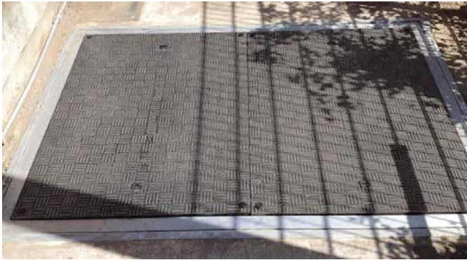
Sealed odour-tight covers installed
