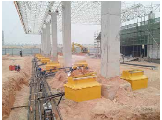
Fibrelite's Gilbarc/China EL-GC-T05403-SH10 dispenser sumps
