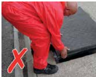
Dangerous lifting technique without Fibrelite lifting aid
