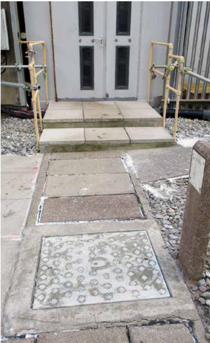
The load capacity of the concrete covers was unknown and thus unreliable
