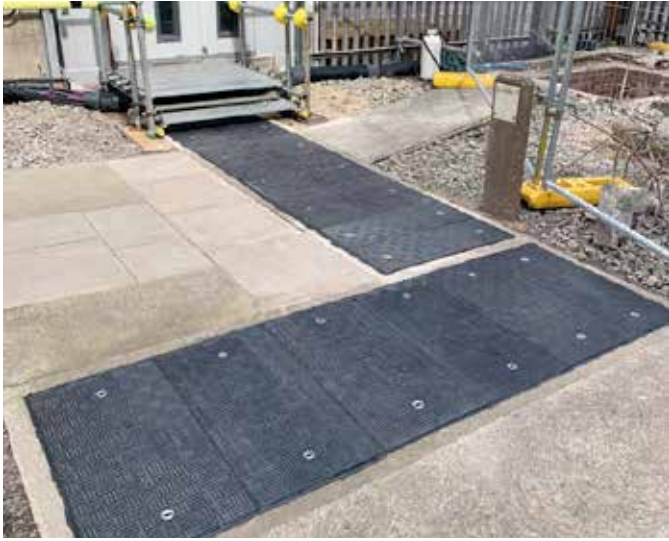
Fibrelite engineered bespoke retrofit GRP trench covers for the Hinkley Point (A) Nuclear Power Station, currently under decommissioning
