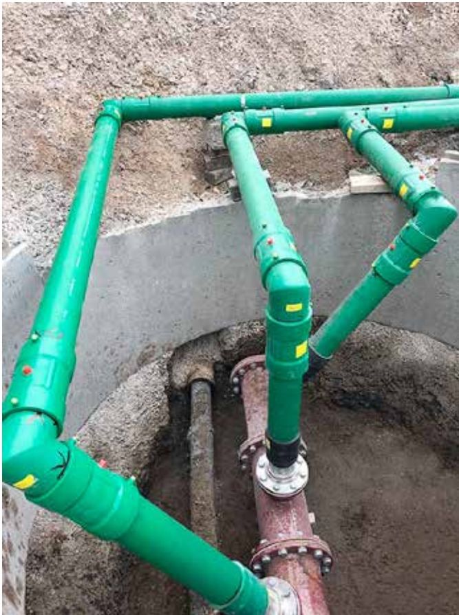
Compact moulded elbows make the join from new KPS piping to the previously installed fuel piping
