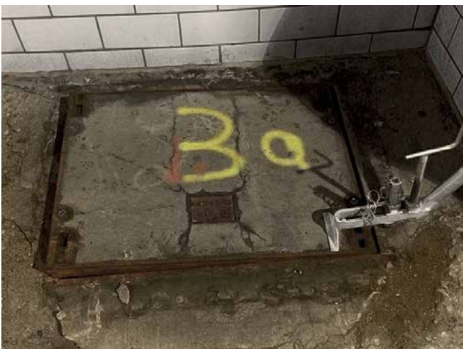
Old unsafe concrete covers
