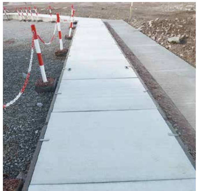
Concrete covers unable to withstand pedestrian traffic
