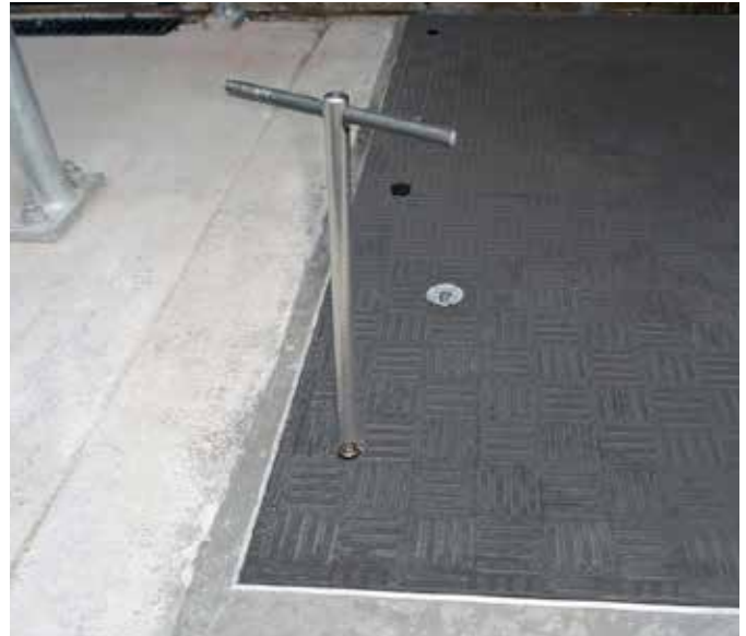
Secured/restrained covers, preventing unauthorised access
