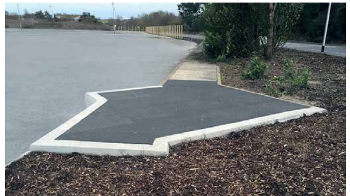
Standard Fibrelite tread pattern provides anti-slip for safe pedestrian traffic
