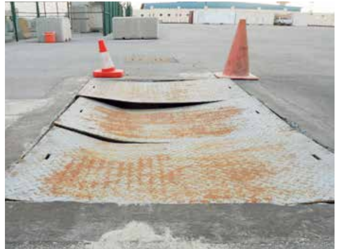
As a result of deformation and corrosion of the covers, dust and debris were entering the trench
