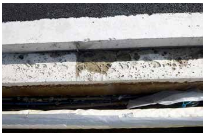
Custom sized covers were required to fit the unusual shape of the trench
