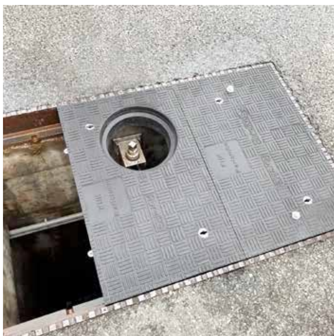
Custom Fibrelite covers retrofit into existing frames, including an inspection port exactly over the slider
