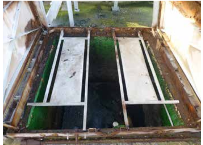
The old heavy mechanical steel covers were replaced with the Fibrelite lightweight alternative
