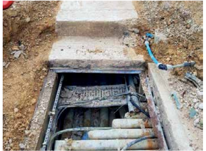
Concrete covers posed a risk of injury to maintenance workers due to their weight
