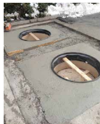
Fibrelite installations are simple – a fiberglass skirt can be used as a preform and to set the frame at grade
