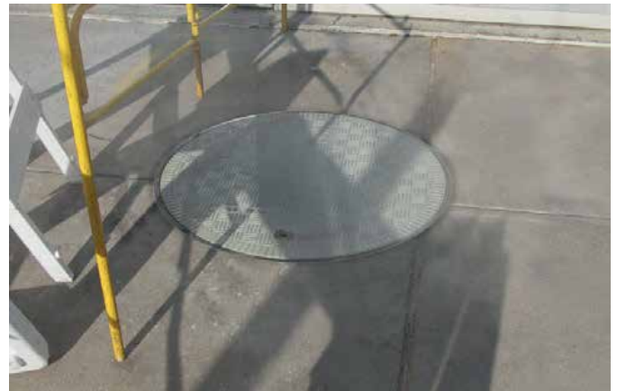
Fibrelite F95 composite cover installed in frame
