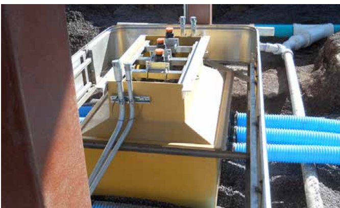
Fibrelite's E85 compatible Encore 500 dispenser sumps
