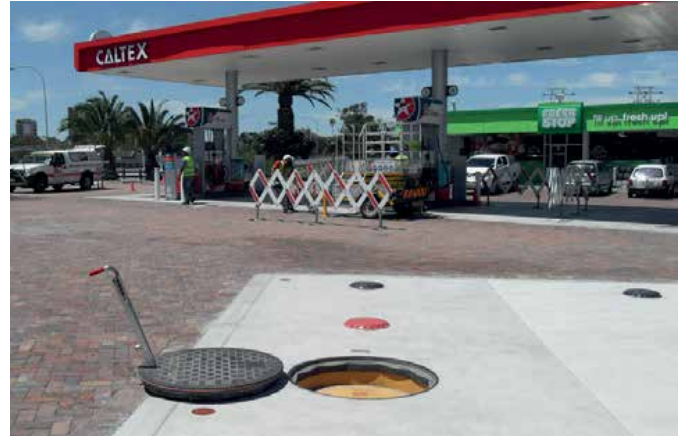
Watertight Fibrelite covers and tank sumps
