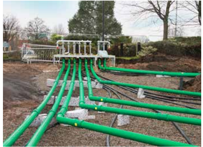
KPS formed bends below fill point
