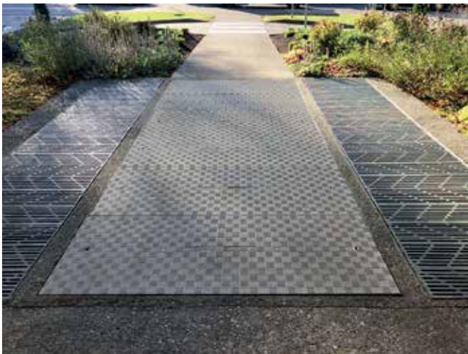
Fibrelite covers allow quick safe manual removal
