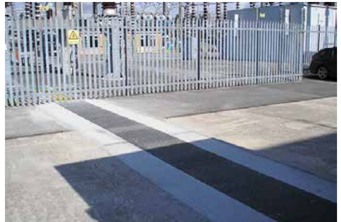
The EN 124 D400 tonne load tested lightweight covers
