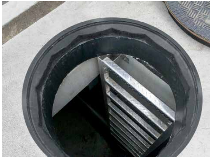
View from over the manhole
