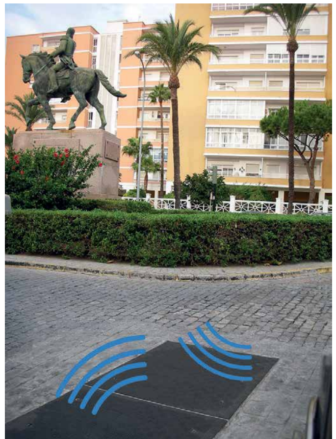
Fibrelite FM45 covers installed allowing RF signals to pass freely through (Image credit: Aguas de Cádiz)
