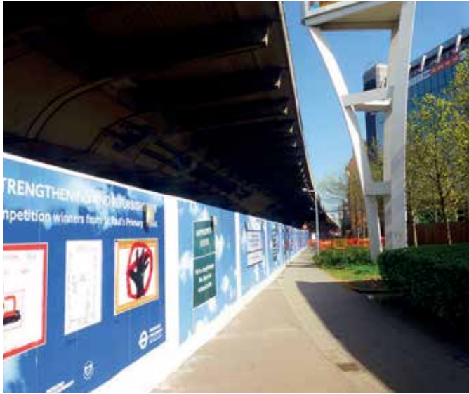
London Hammersmith flyover during refurbishment
