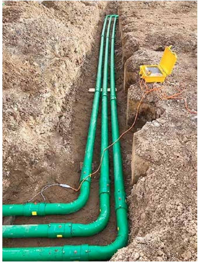
KPS double wall diesel piping
