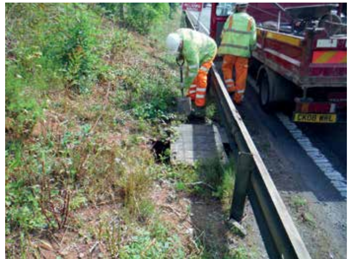
Heavy covers present a hazard for operators
