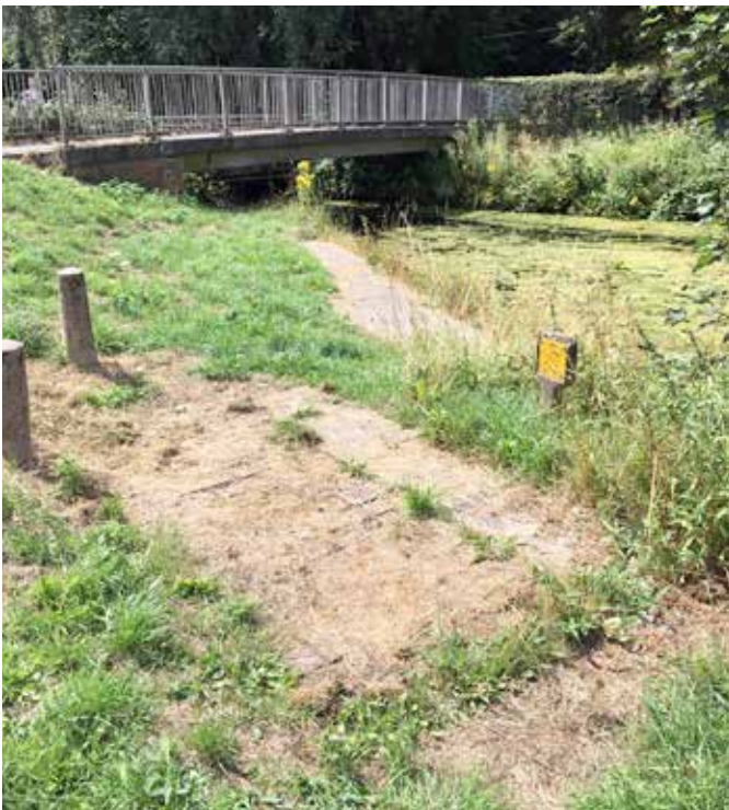
Previously installed covers had begun to degrade/rust
