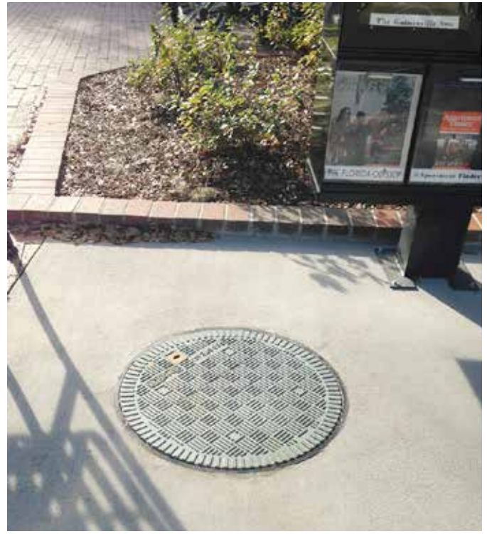
Lightweight composite steam cover - product code F65
