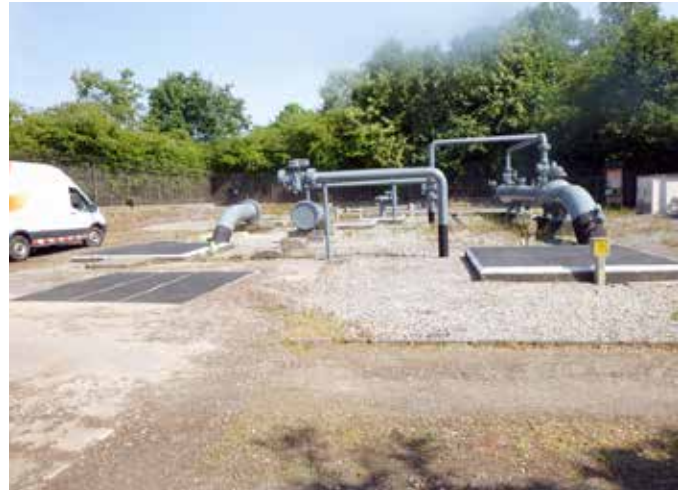
A custom covering solution was required to fit existing apertures and accommodate piping entering trench
