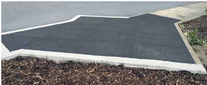
Bespoke "cassette" of Fibrelite covers and supporting steelwork installed to tight construction deadline
