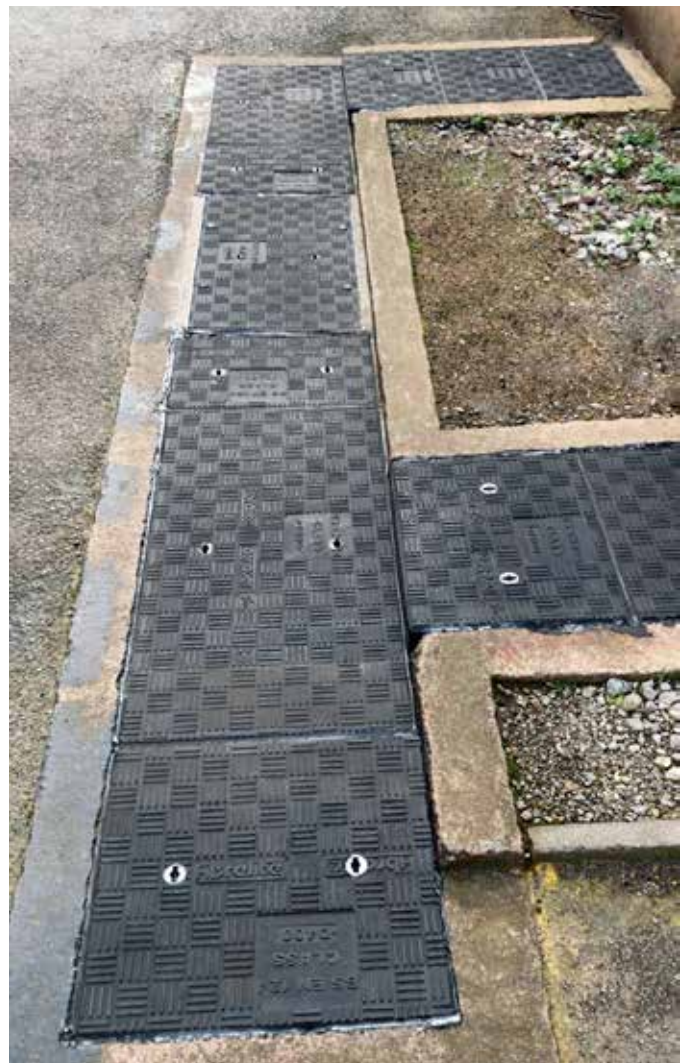
The nuclear facility now has a safe covering for their utilities during the decommissioning work
