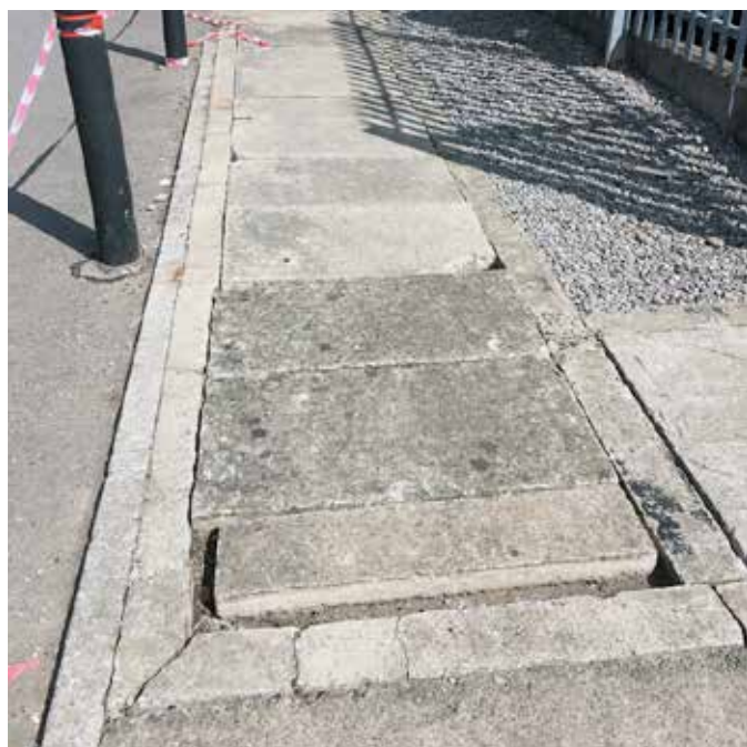
Previously installed failing concrete trench access covers
