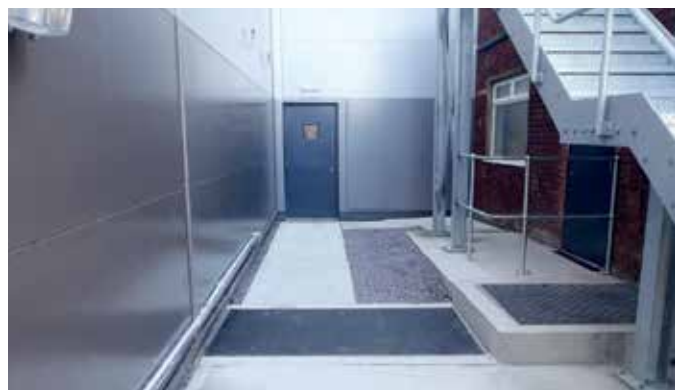
Retrofitted sealed Fibrelite covers installed
