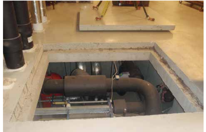
The geothermal monitoring pit
