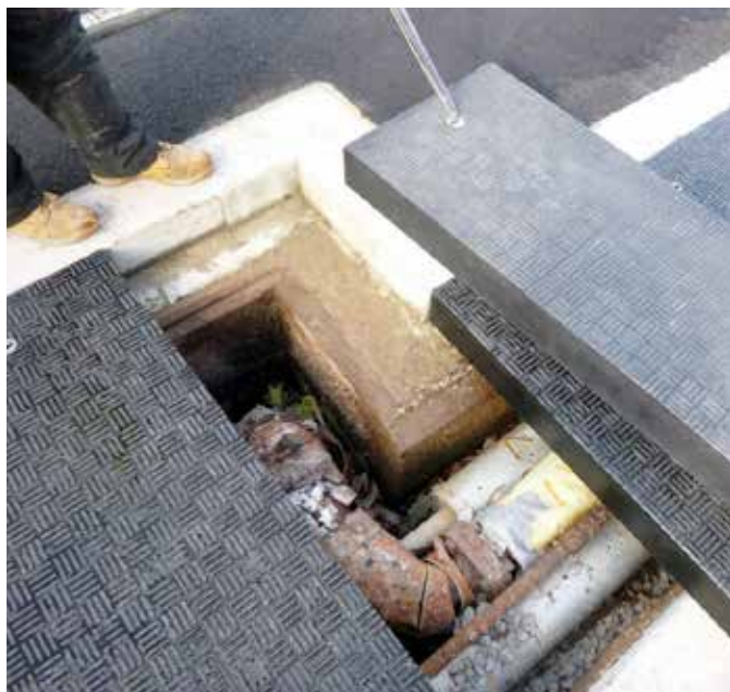
The scale and requirements of this project necessitated a carefully planned bespoke design
