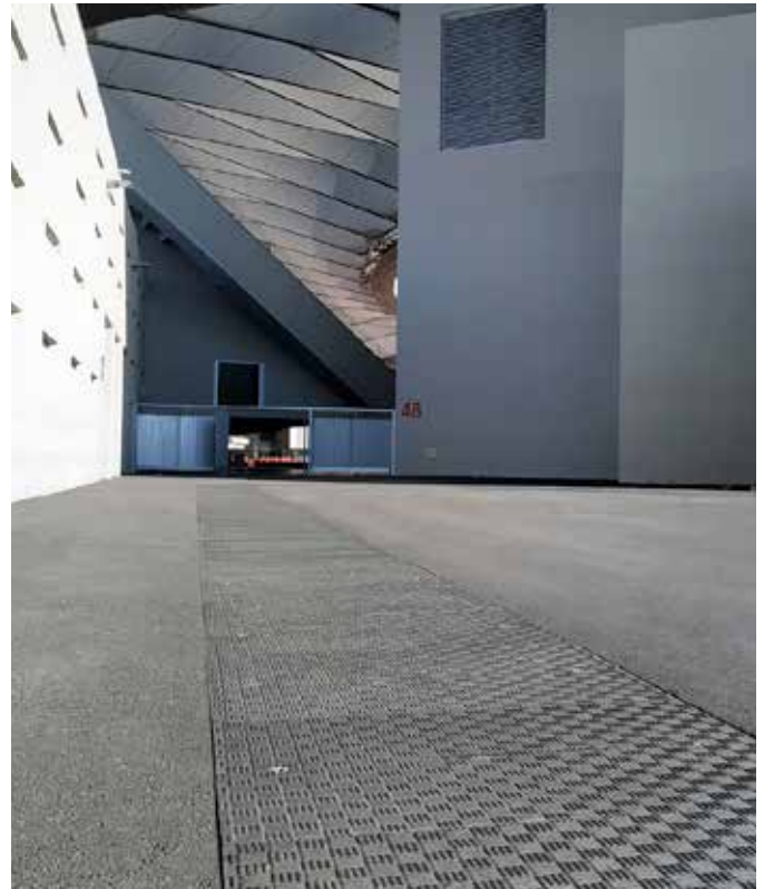
This project was completed within 2 months of the official PO
