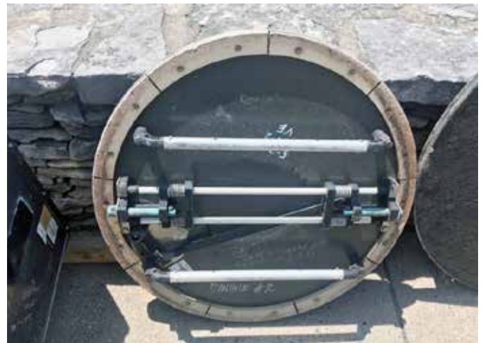
The adverse conditions of the steam vaults had caused the locking mechanisms to fail
