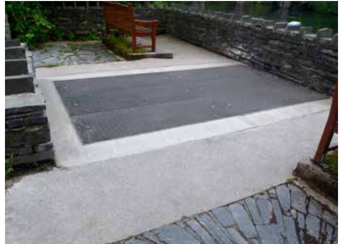
Lightweight Fibrelite trench covers now installed
