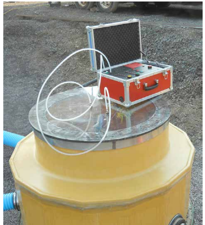
Vacuum testing to ensure a watertight installation
