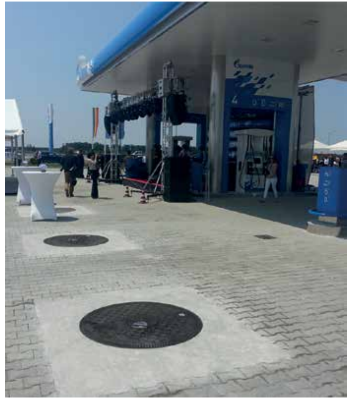
Fibrelite's FL100/CD cover. The central dip cover makes it easy to access the riser without having to remove the whole cover
