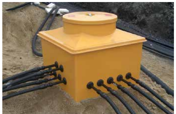
Fibrelite's electrical conduit drawpit being installed
