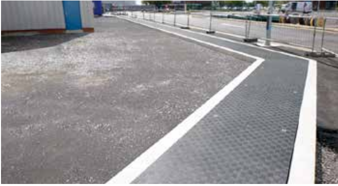
Fibrelite covers are chemically inert
