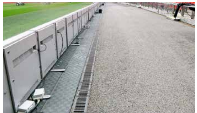
Lightweight Fibrelite covers allow easy, safe removal by 2 people
