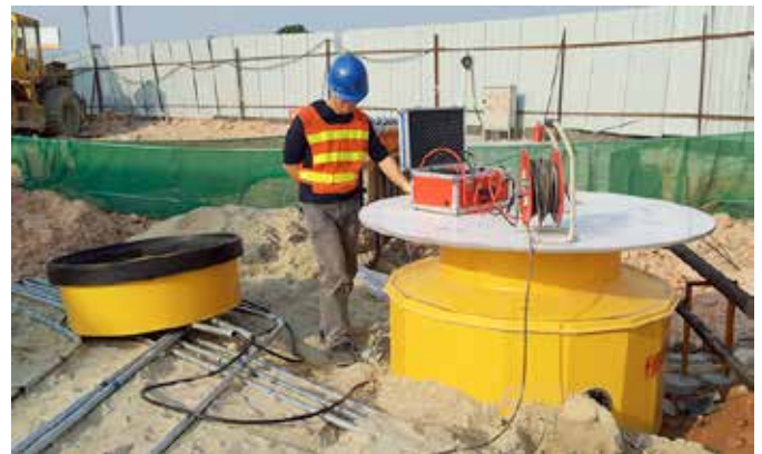
Vacuum tested tank sumps
