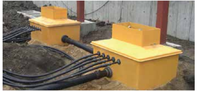
Fibrelite's Tokico AB26L dispenser sumps
