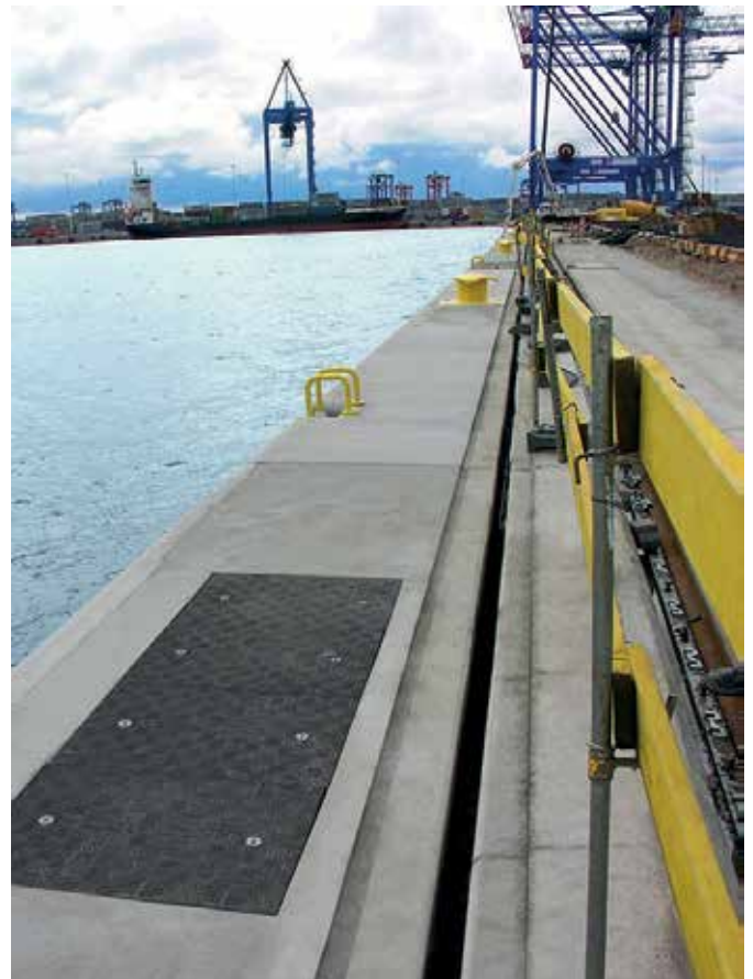
Fibrelite's trench covers covering access pit
