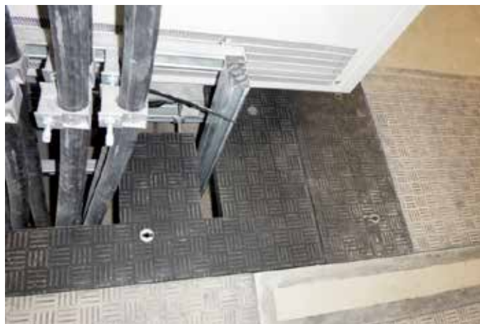
Custom Fibrelite trench access covers designed with cut-outs to accommodate piping and cabling
