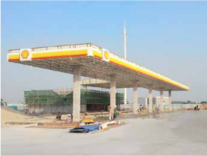
Site under construction
