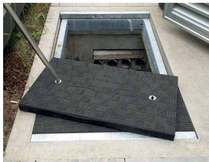
Fibrelite trench panels installed over the chamber
