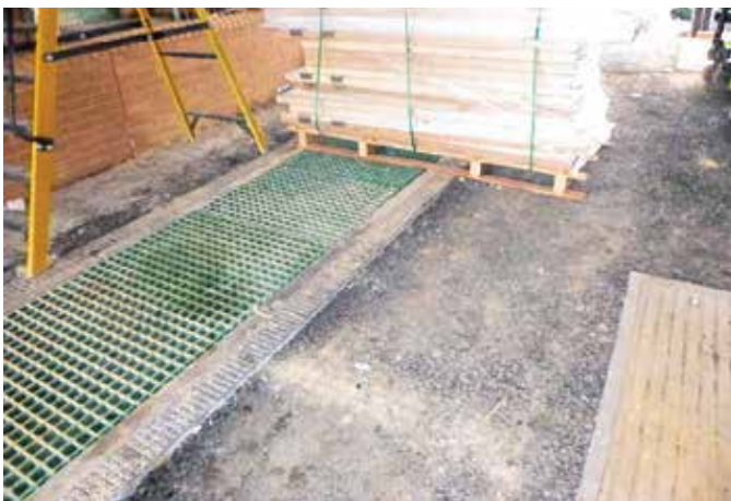
Previously installed GRP grating was originally supplied together with the precast concrete troughs
