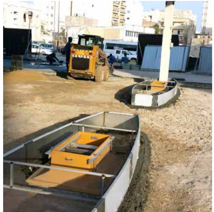
Fibrelite EL-G-E500 dispenser sumps ready for concreting
