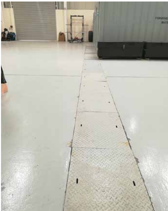
Previously installed steel covers
