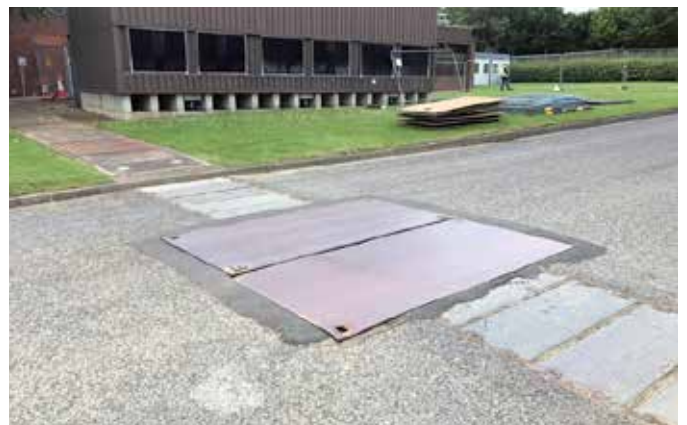
Sheets of metal had been installed as a temporary patch over failing concrete covers
