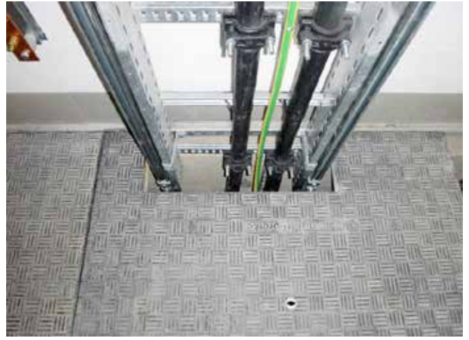
This project had an extremely tight timeline to minimise disruption to the facility
