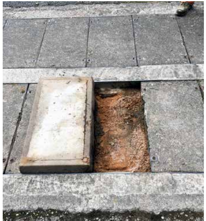
The previously installed covering arrangement was deteriorating
