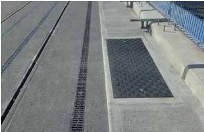
Bespoke trench covers for trackside gear
