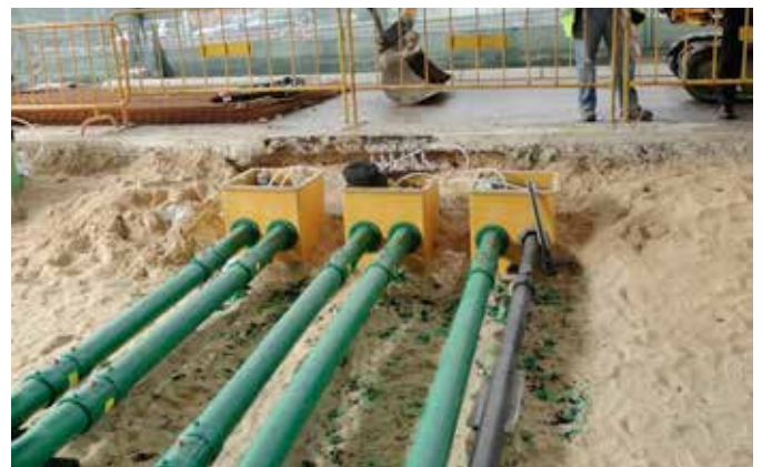
Fibrelite remote fill sumps and KPS conductive double wall fill pipe
