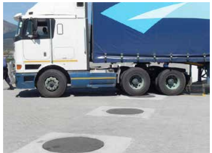
Fibrelite cover installed in truck lane
