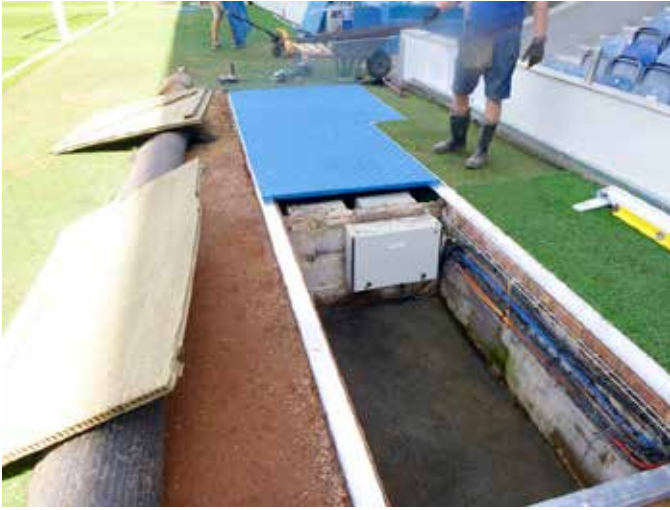
Fibrelite installed a range of lightweight covers which can be removed and replaced by two people using the ergonomically designed FL7 lifting handles
