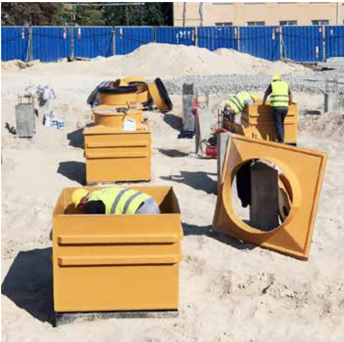
Technical support and installation training was required on site to complete the project within its tight timescale
