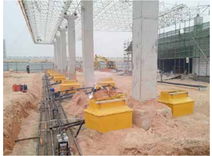
Fibrelite's Gilbarc/China EL-GC-T05403-SH10 dispenser sumps
