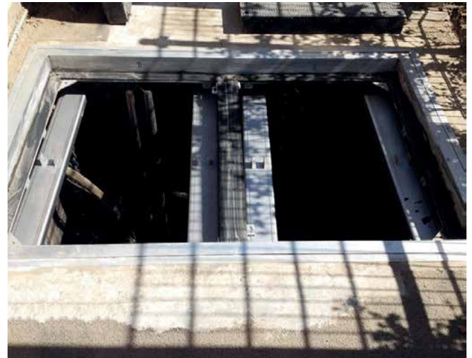
Removable centre beam supports covers
