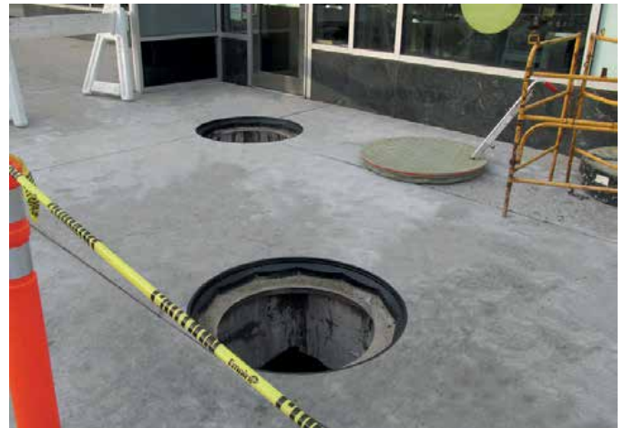
Fibrelite F95 composite cover installed in frame
