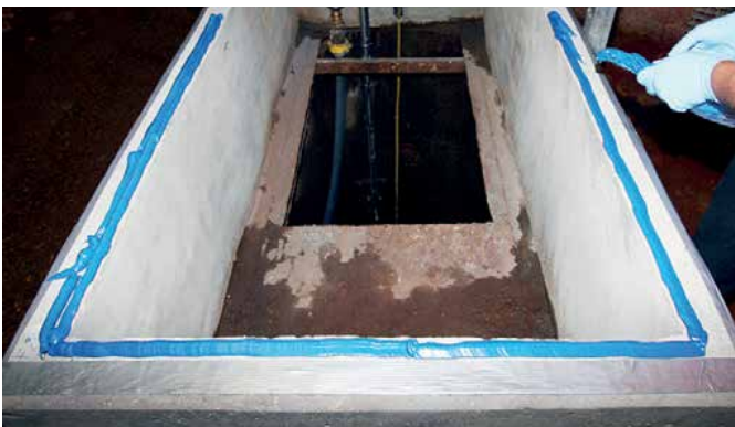
The blue epoxy resin is applied to the base
