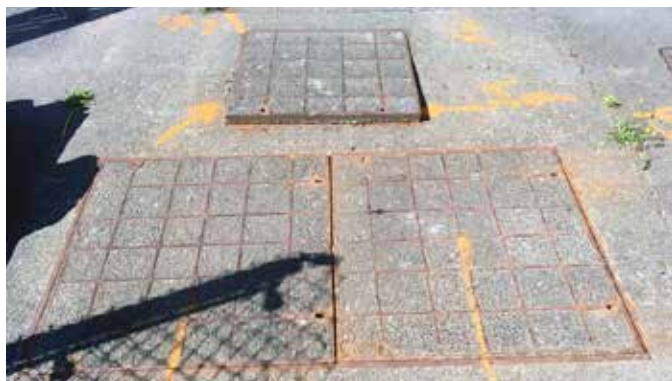
Covers were showing signs of severe corrosion
