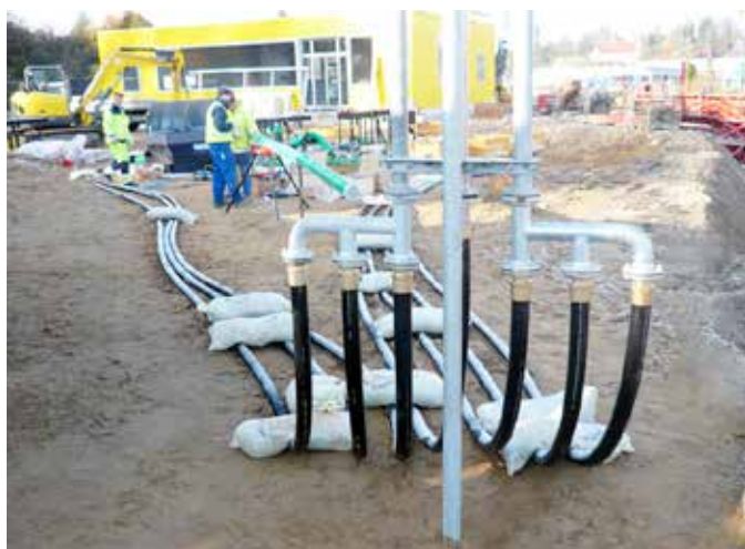
KPS semi flexible pipe system is unaffected by earth movements
