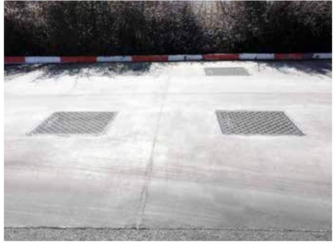
Fibrelite watertight manhole covers helped LUKOIL to eliminate water ingress
