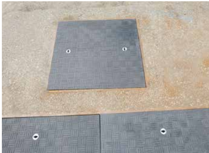
Covers were manufactured to fit existing frames
