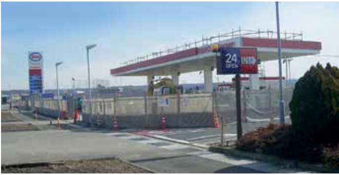
Site under construction
