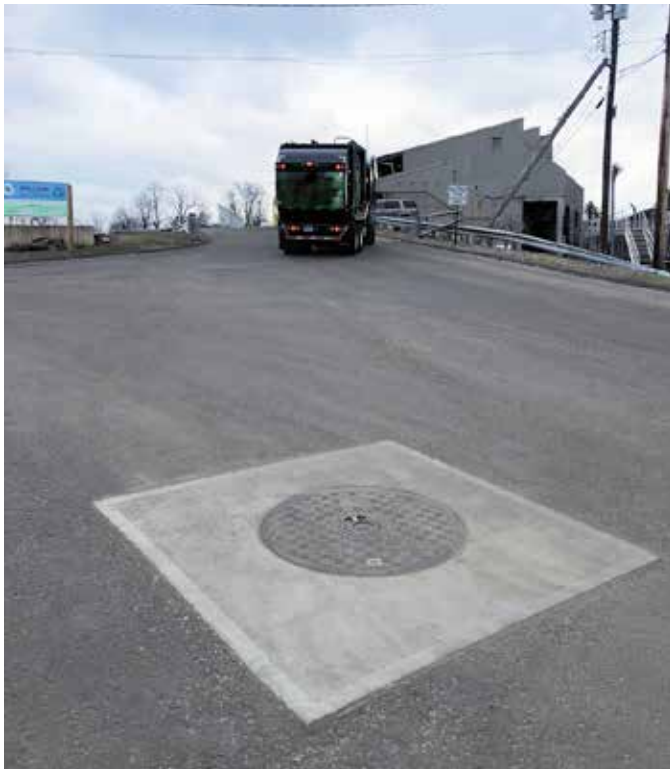
This water company contacted Fibrelite about the possibility of installing automatic water meter readers in or beneath a composite cover
