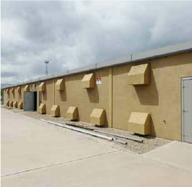
UK gas valve plant
