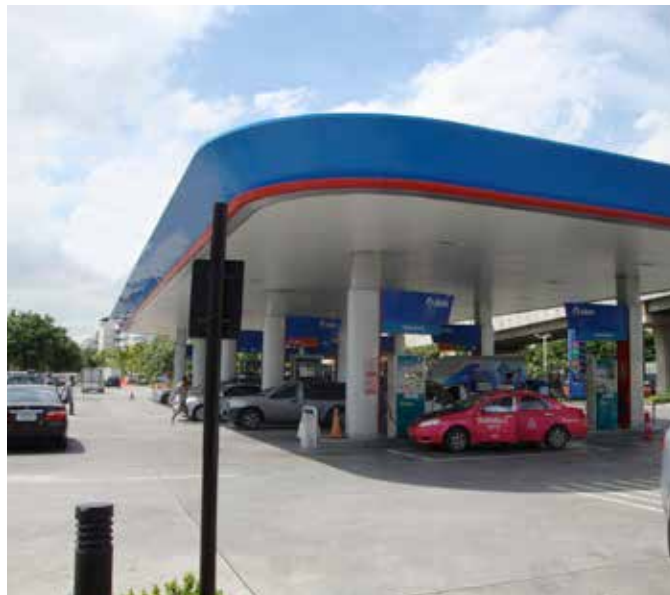
Thailand Petrol Forecourt and Green Area
