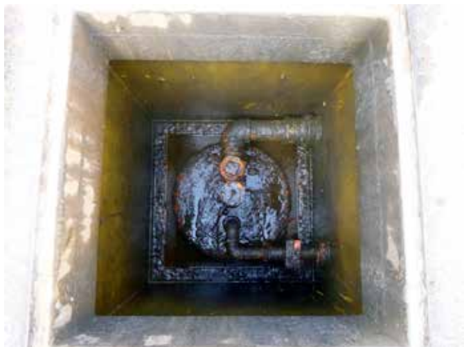
Previously installed chambers allowed water ingress
