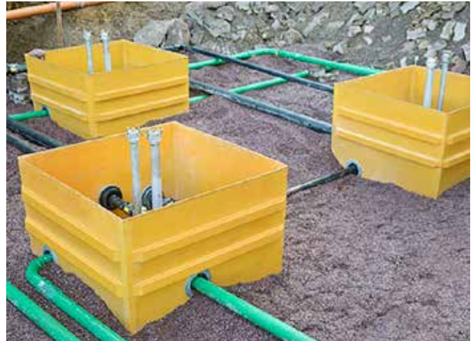
When the first site was under construction, the OPW team were on hand to offer onsite installation and guidance
