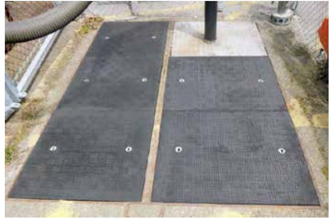
Fibrelite covers allow safe removal by hand
