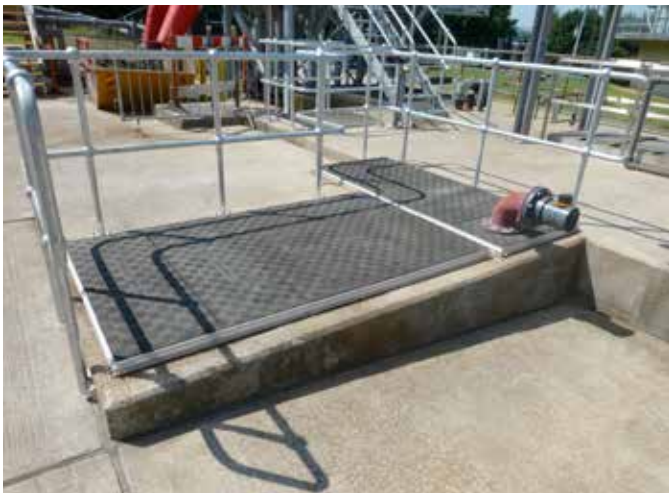
Specialised vent pipe could also be incorporated into the Fibrelite design
