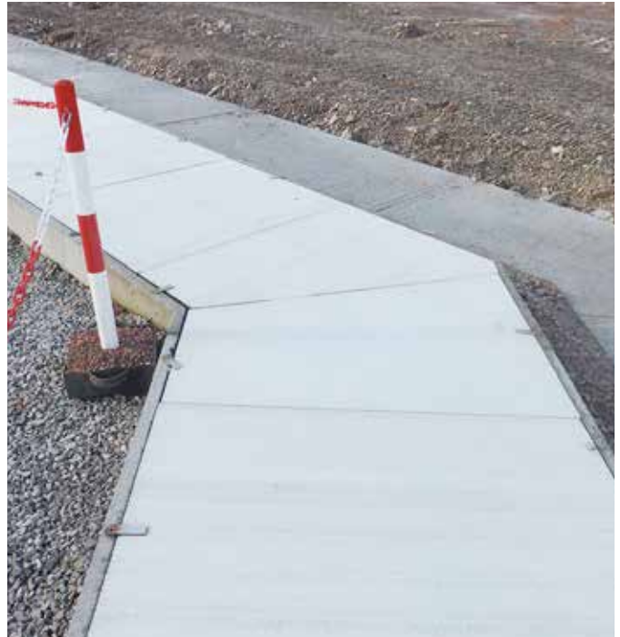
Previously installed low quality concrete covers
