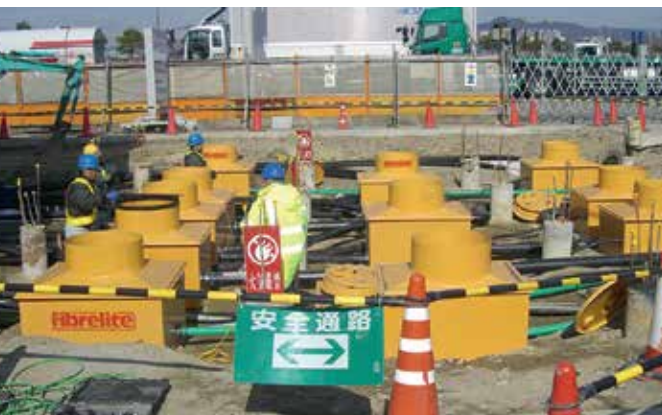
Vacuum tested tank sumps
