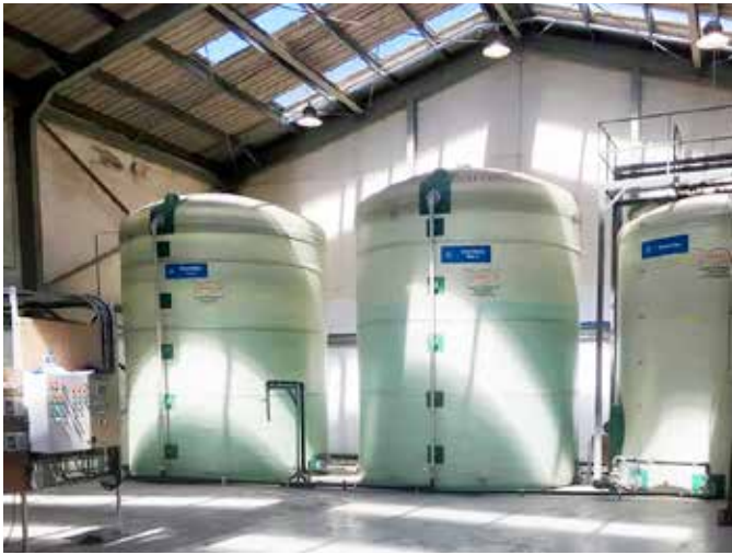
KPS piping proved the perfect solution for this new Maxol AdBlue production facility
