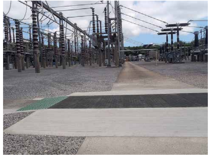
Covers are non-metallic, non-conductive and will not spark
