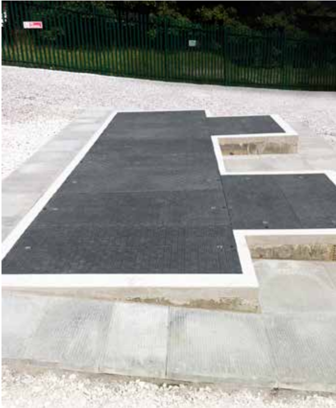
These bespoke trench covers were custom designed to offer easy access to the entire trench
