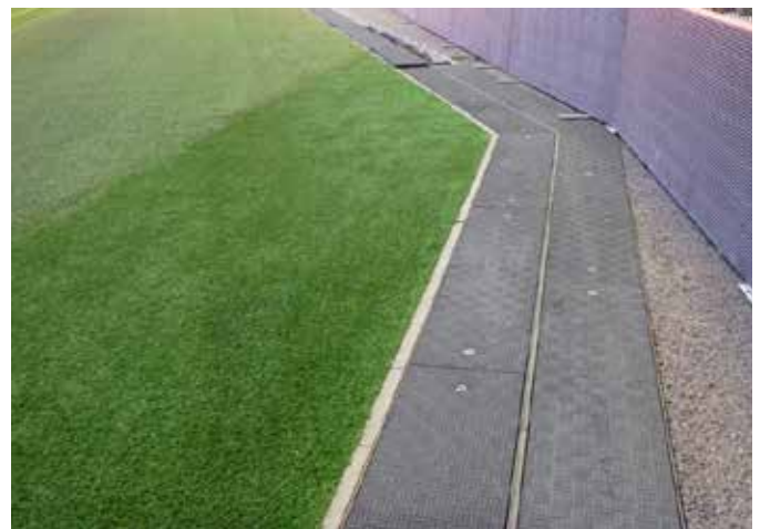
Fibrelite covers provide a superior anti-slip surface in both wet or dry conditions
