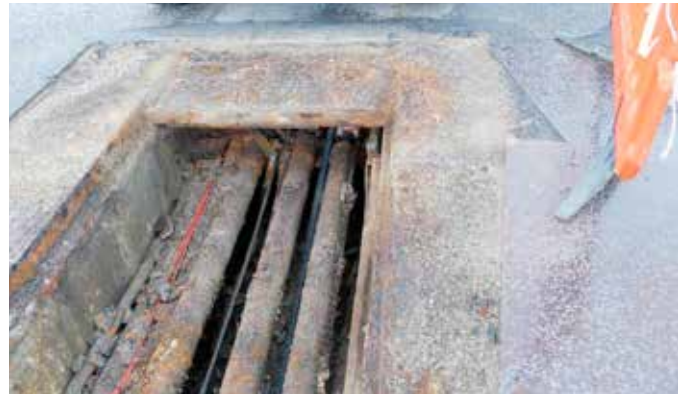
Previously installed failing concrete and metal covers
