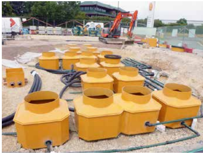
Bespoke Fibrelite chambers installed at Shell Eastfield
