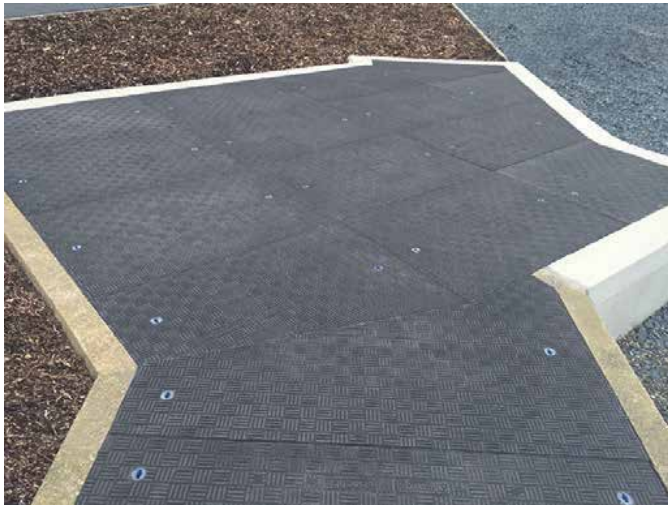
"Cassette" of bespoke covers over culvert
