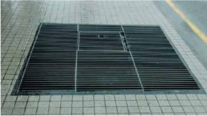
Metal covers causing a trip hazard for pedestrians
