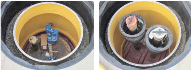
Fibrelite turbine and fill sumps
