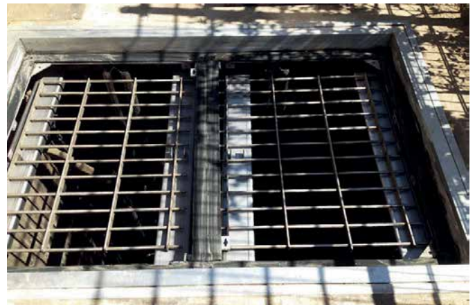
Removable beams hold safety grid
