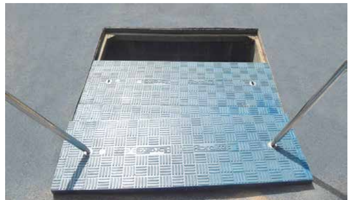
The recently installed Fibrelite coloured trench covers
