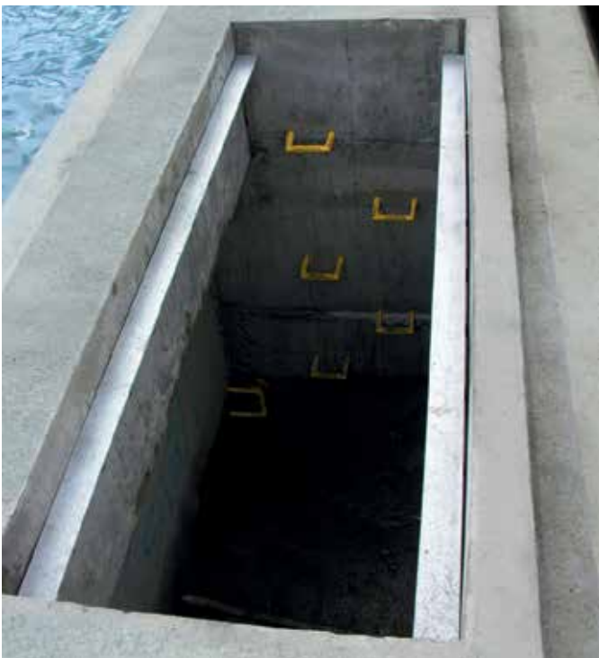
Access pit along edge of quay
