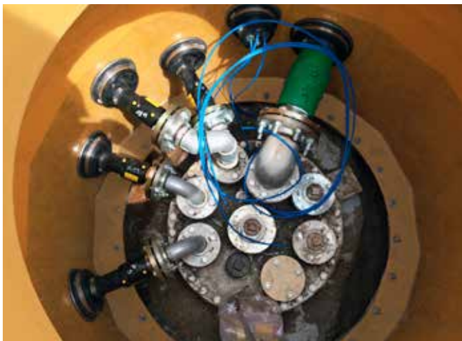
OPW provided a long-lasting containment system
