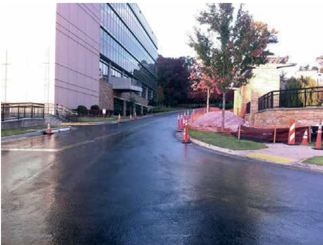
Pre-install location for the Fibrelite covers
