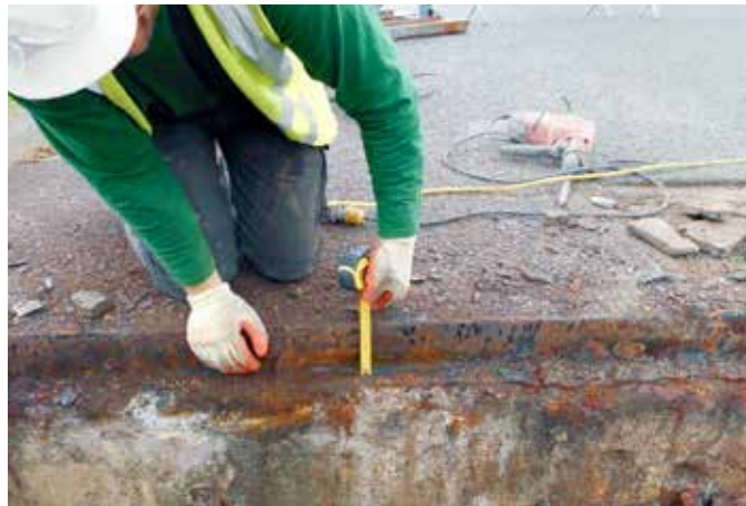
Previously installed heavily corroded access covers
