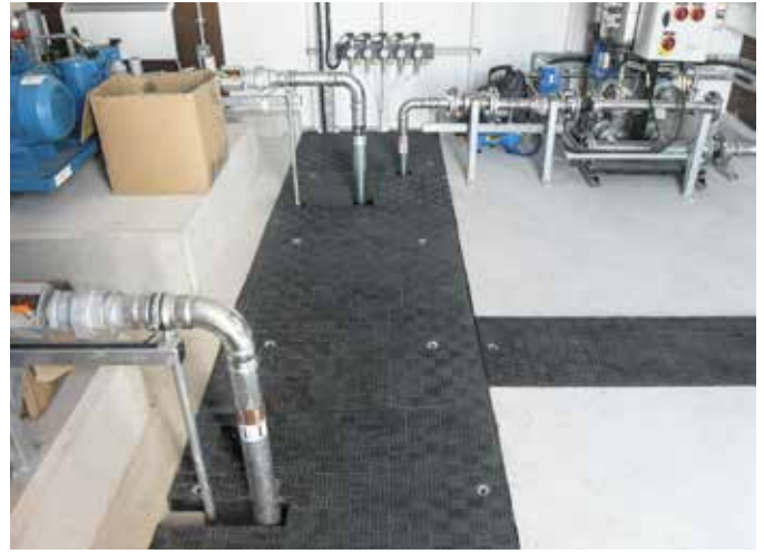
Fibrelite covers can accommodate service pipes of all shapes and sizes
