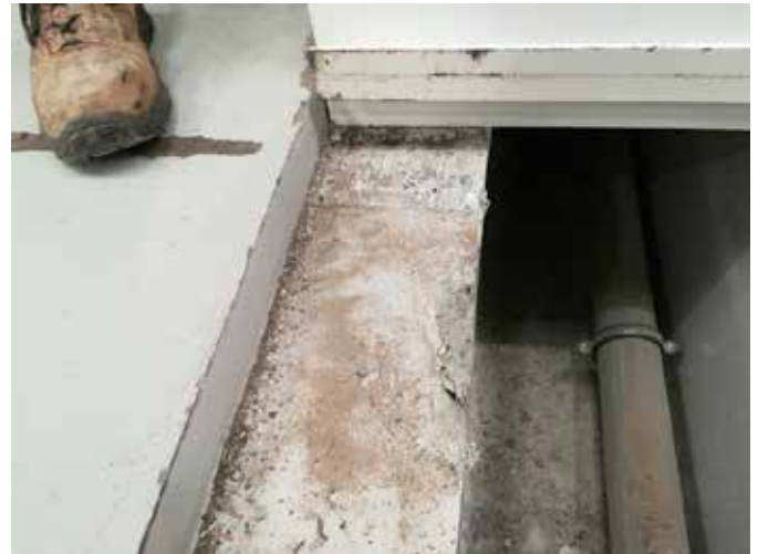
Uneven trench recess depth
