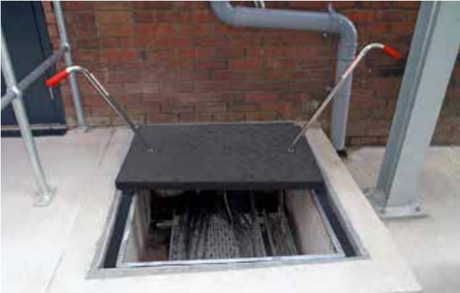
Sealed Fibrelite covers prevent water ingress
