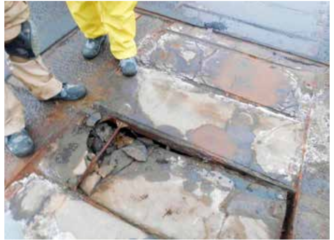
Heavily corroded previously installed covers
