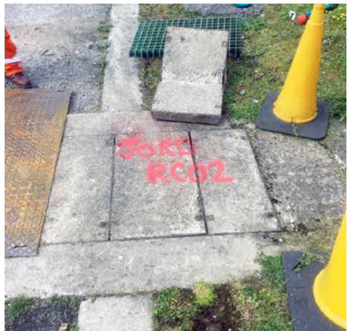
Covers were extremely heavy to lift
