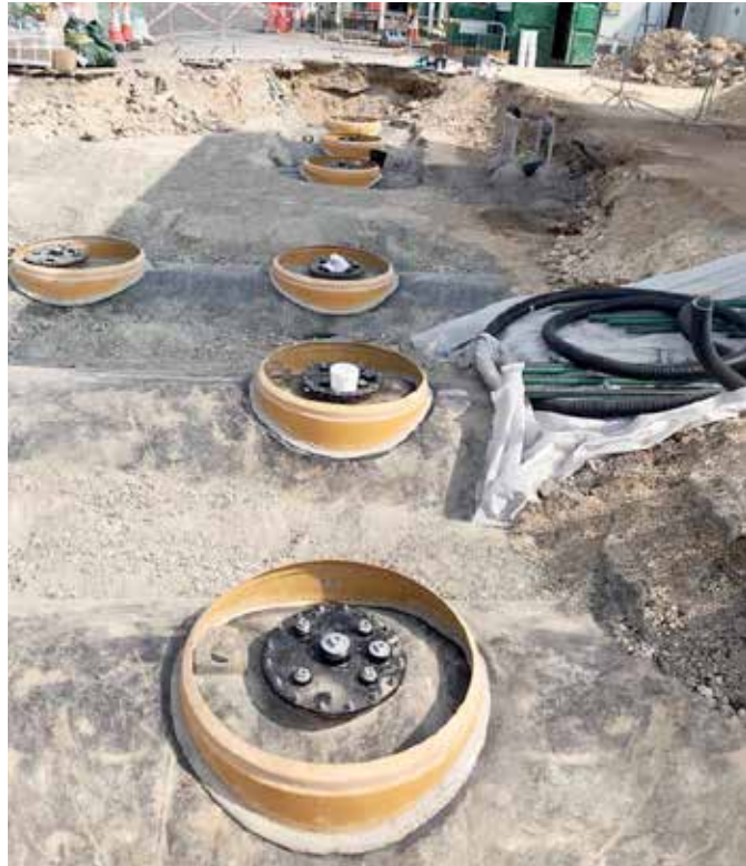
Fibrelite collars bonded ready for chamber installation
