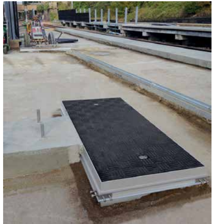
Fibrelite FM45-B125 trench cover
