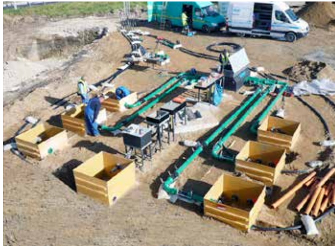
Fibrelite tank sumps and KPS piping provide a complete secure system
