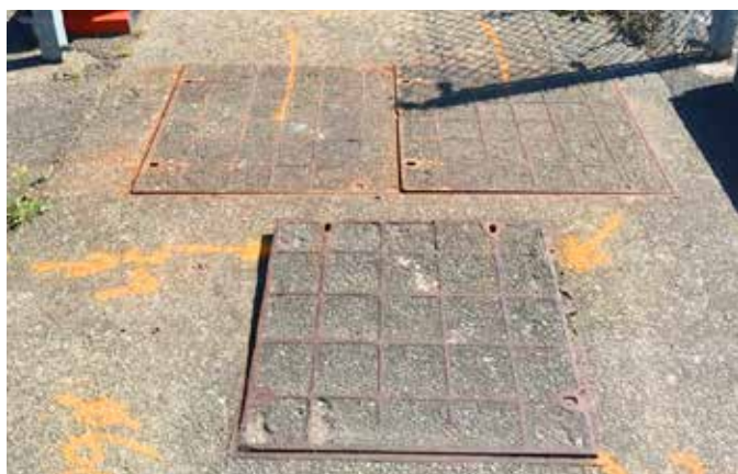
Previously installed heavy concrete recess covers
