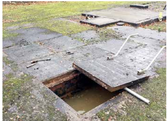
Previously installed covers were extremely difficult to remove and replace safely
