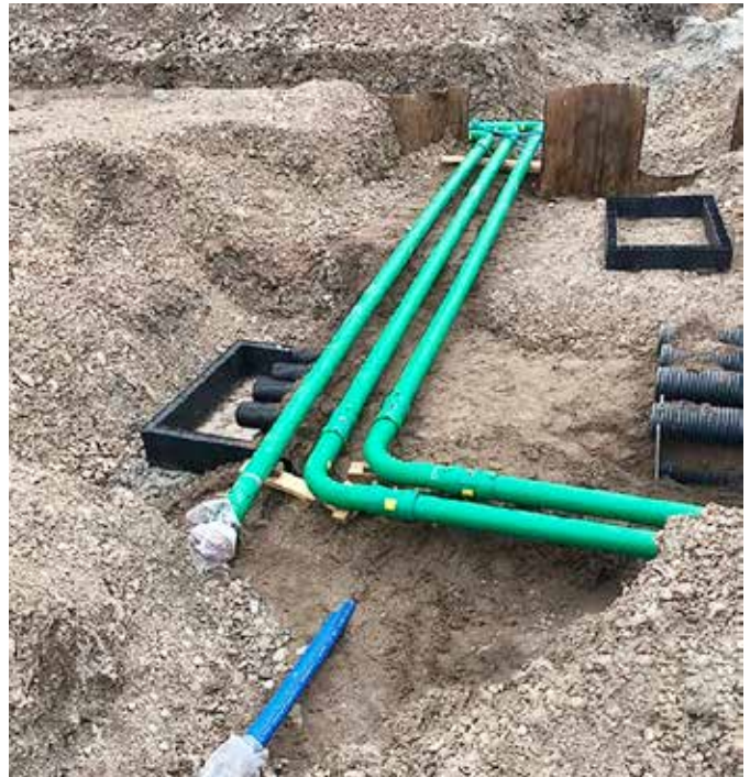
KPS double wall piping, allowing monitoring of interstitial space
