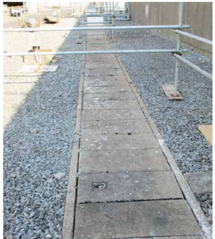
Exclusion zones were put in place to prevent loading causing a failure of the covers during the decommissioning work
