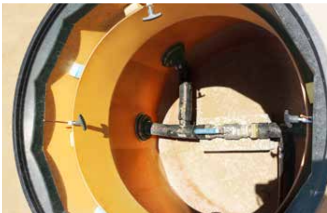
Vacuum testable Fibrelite pipe sealkits form watertight seal
