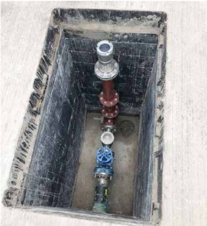
Complete below ground remote fill point
