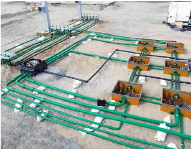
KPS piping had to be installed within 5 working days to meet the strict project deadline
