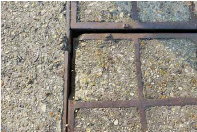
Corroding previously installed covers
