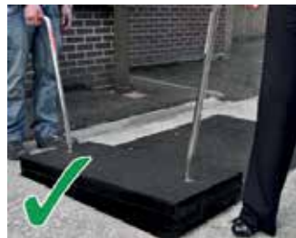
Safe lifting technique with Fibrelite Lifting aid
