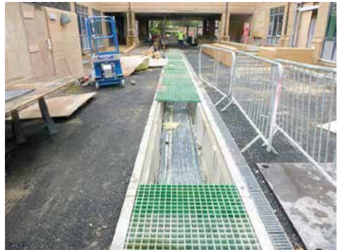
The client required a higher performance replacement
