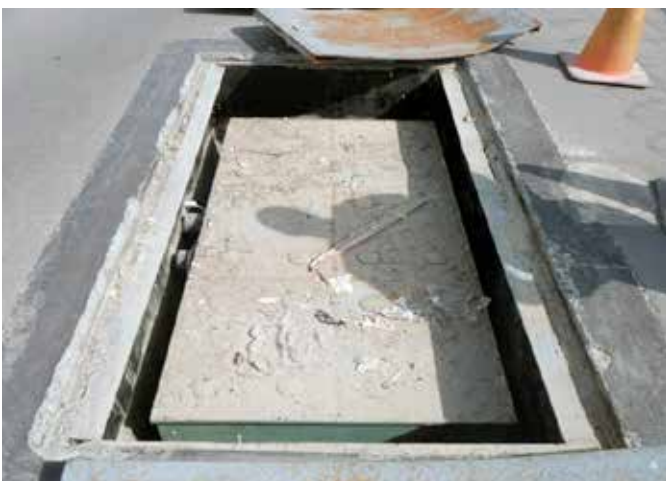
Previously installed chequered metal plate covers had deformed due to HGV traffic
