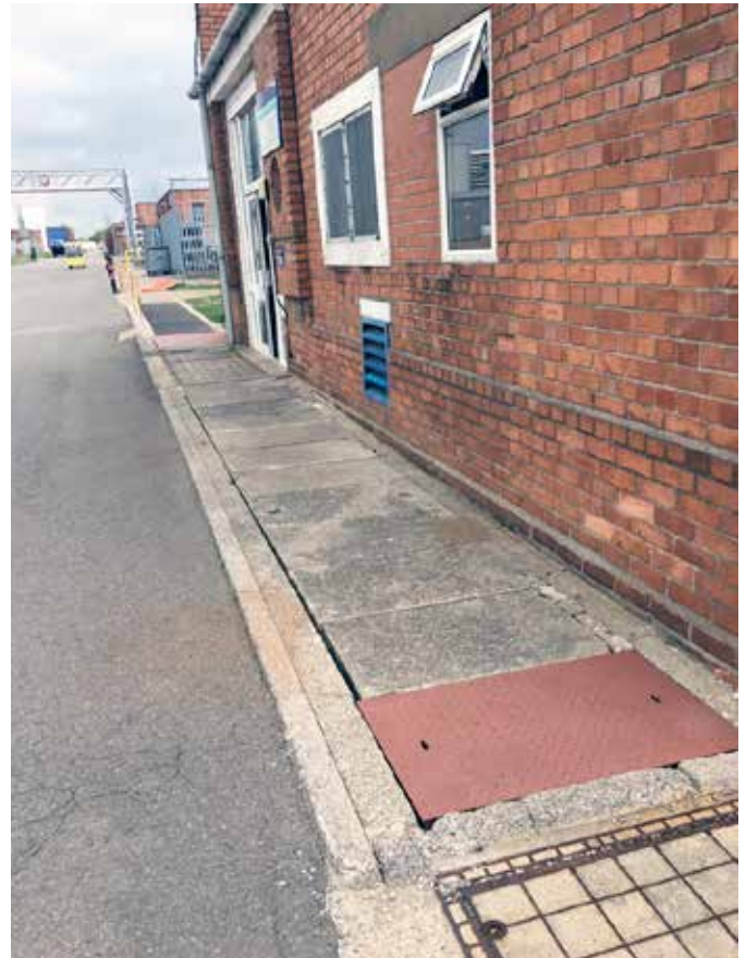
Previously installed covers had cracked and corroded
