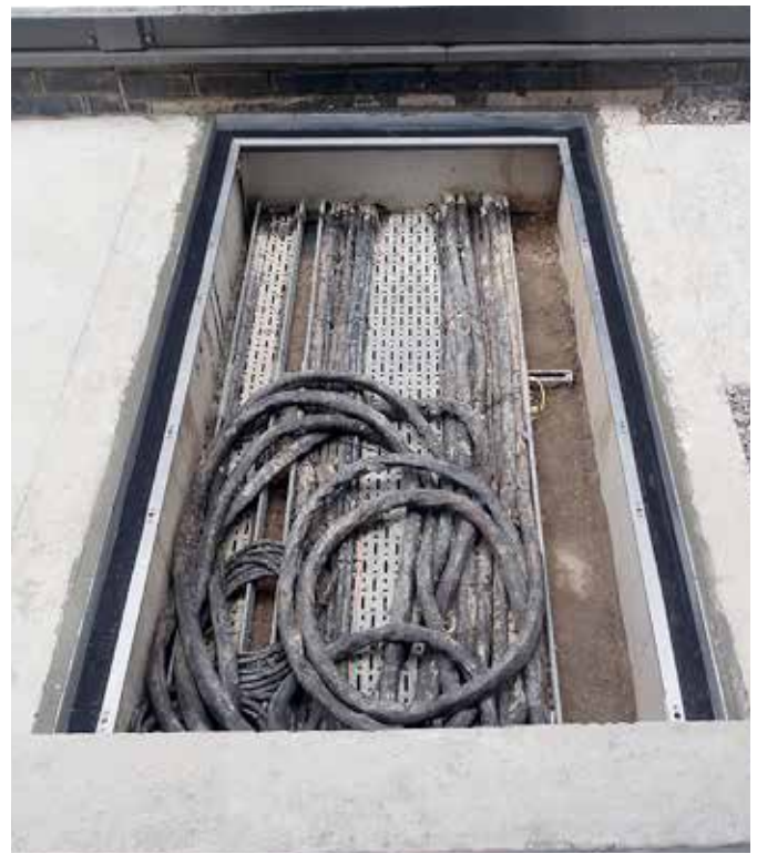
Aluminium frame set into existing steel frame with epoxy grout
