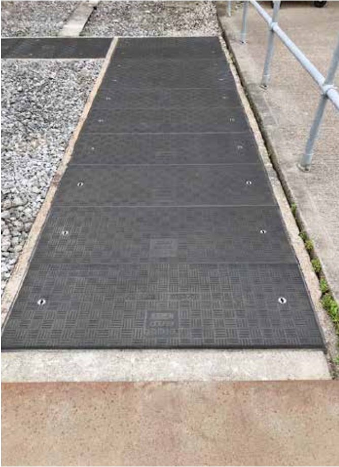
Fibrelite covers are chemically inert and have an anti-slip tread pattern
