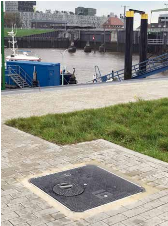
Fibrelite's manhole covers were installed with an additional dip port in the main lid
