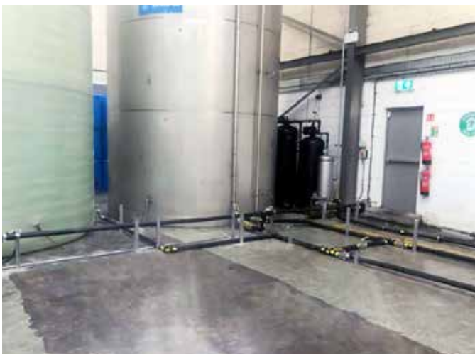
This project had a tight build schedule, so installation time was key
