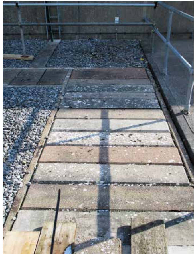
Previously installed concrete trench access covers had begun to corrode
