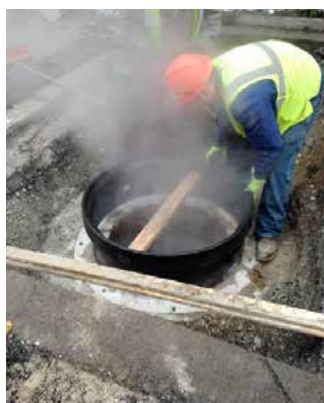
Fibrelite installations are simple – a fiberglass skirt can be used as a preform and to set the frame at grade
