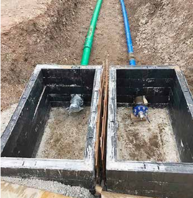
KPS piping provides a zero-permeation solution
