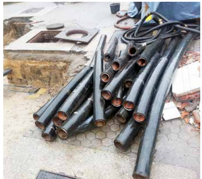
The previously installed steel piping had less flexibility than KPS piping
