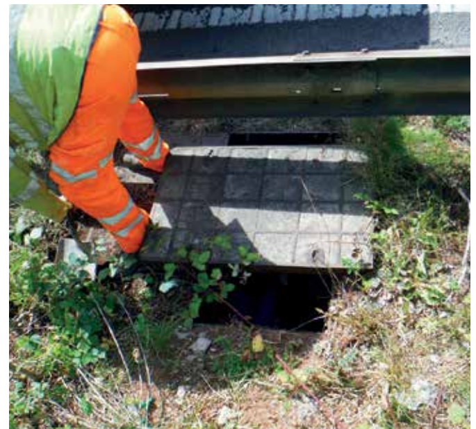
Damaged cast iron and concrete cover
