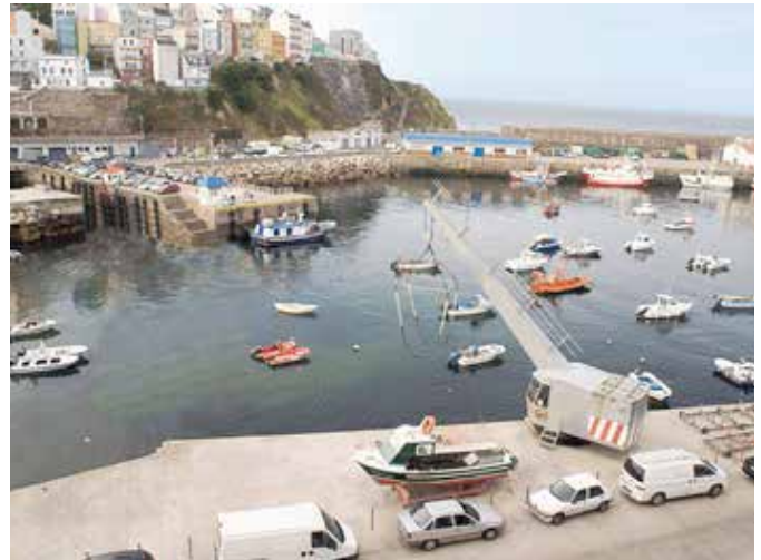
Malpica port now has a safe and reliable piping system thanks to KPS
