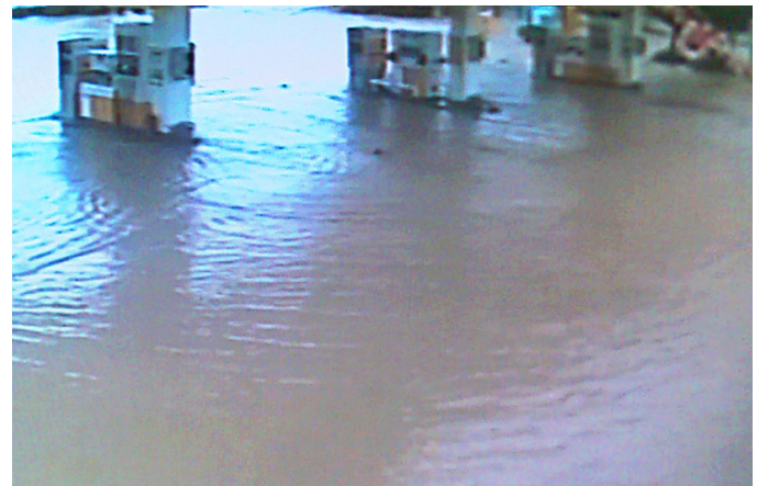
Some petrol stations in Istanbul were submerged during the July 2017 floods
