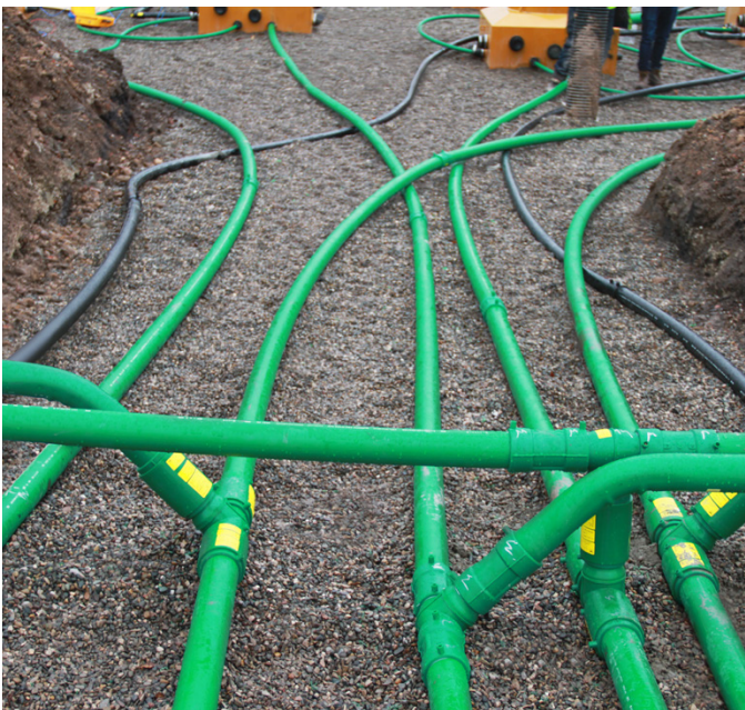
All integrated double wall KPS fittings weld both pipe walls simultaneously
