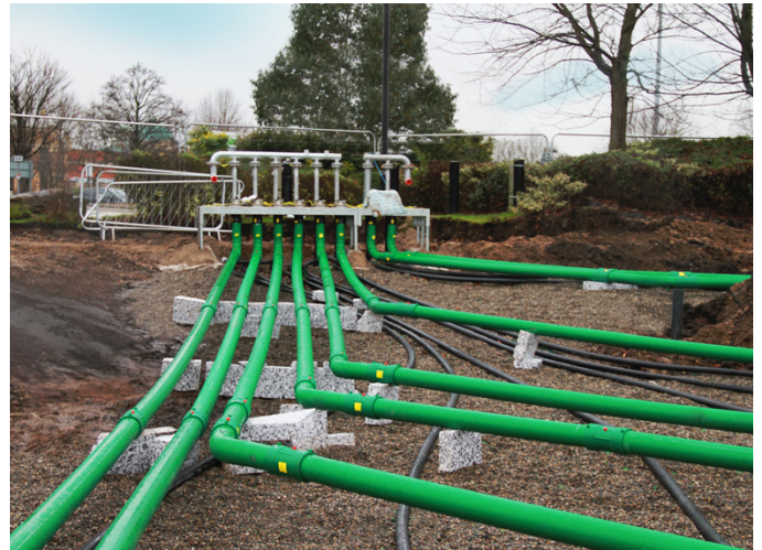
KPS formed bends below fill point
