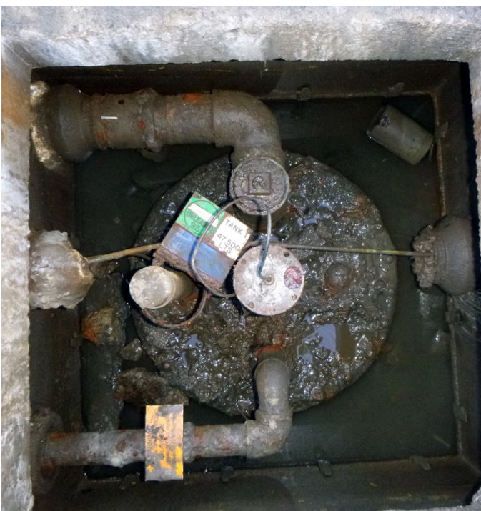
At this site, the old tank upstands were too small for the traditional bolt down tank sumps / chambers
