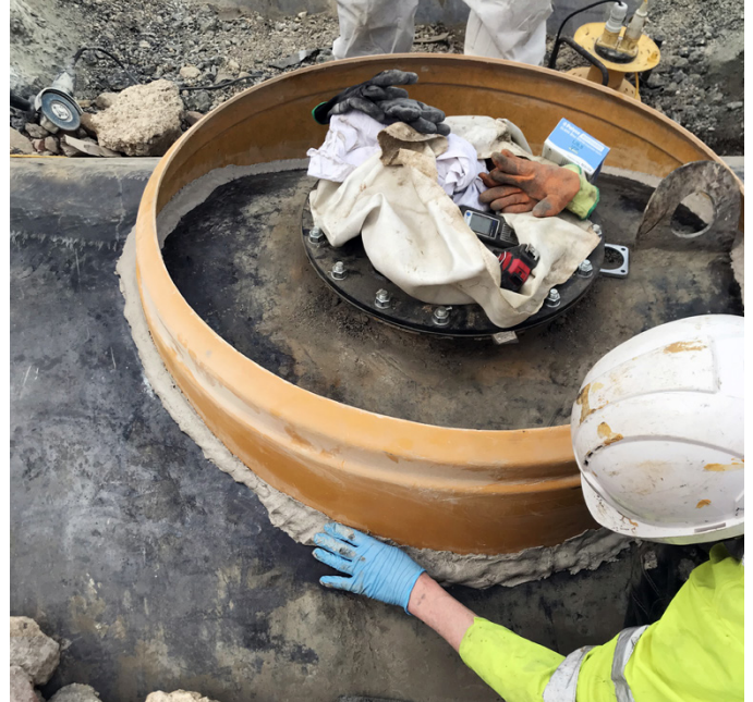
Bonding of the collar to the tank
