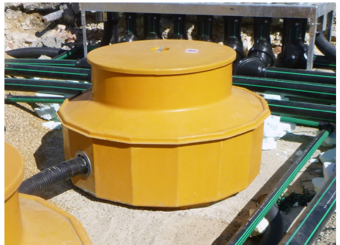
Fibrelite tank chambers were laminated to the collars
