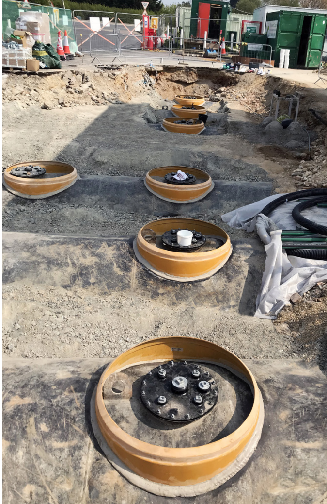
Fibrelite collars bonded ready for chamber installation
