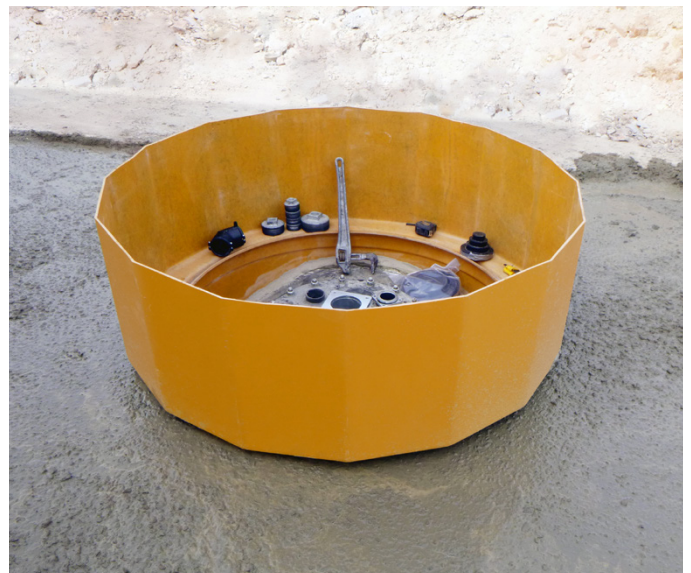
An epoxy putty compound was used to bond the collar directly to the tank
