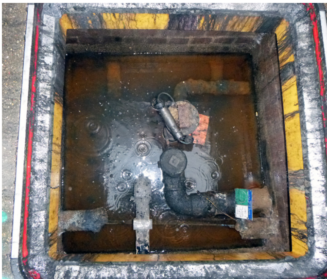
Previously installed brick chambers
