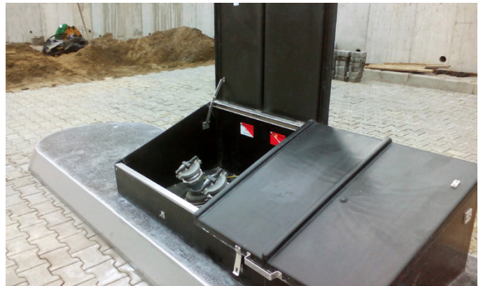
Vacuum testable GRP sump prevents water ingress from above or below ground
