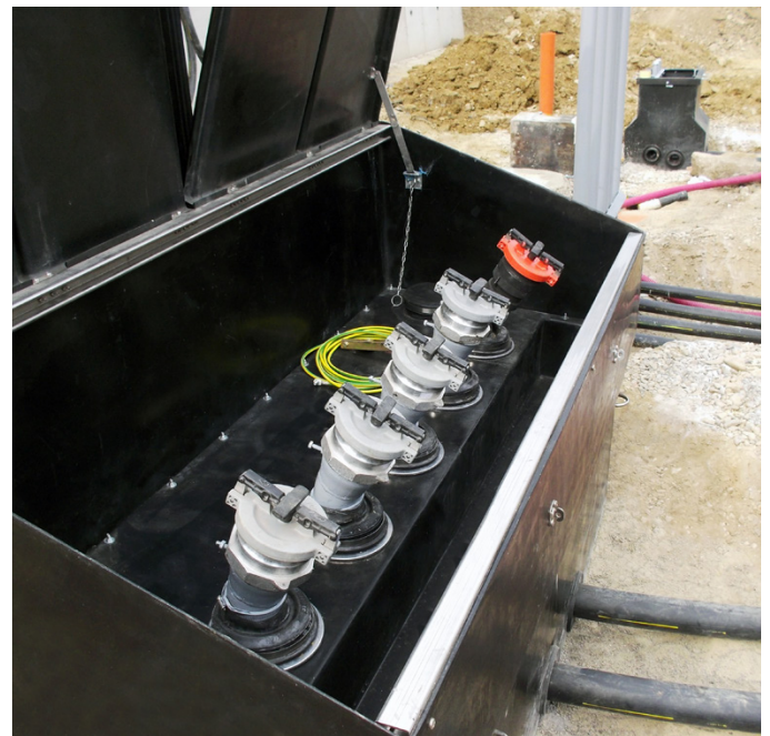
Installer friendly KPS piping used to connect fill points to tanks
