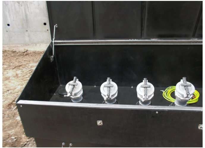
OPW heavy duty corrosion resistant seal caps
