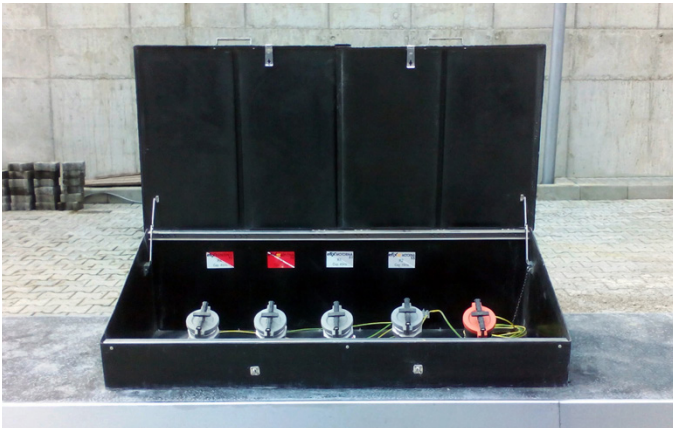
Vacuum Testable Fibrelite GRP Above Ground Remote Fill
