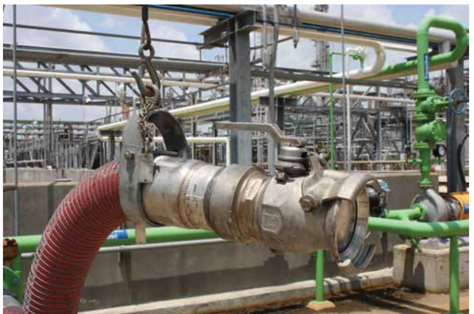
The Drylok dry disconnect coupler
