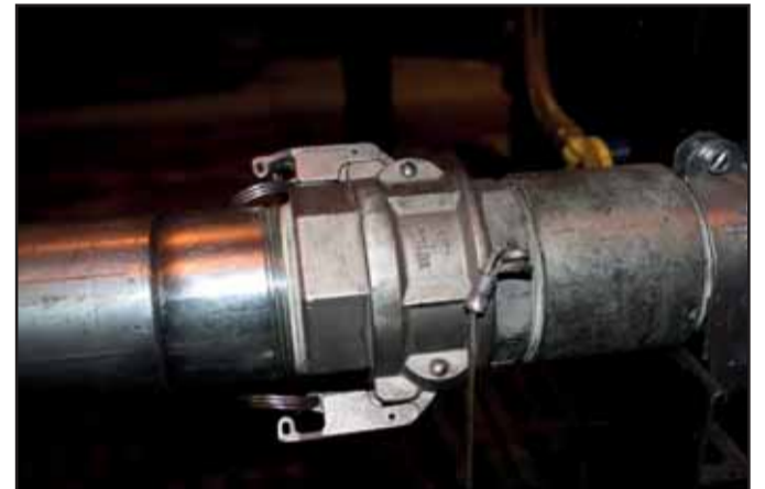
Autolok Quick Disconnect Couplings play an integral role in ensuring the safe and reliable transfer of hazardous chemicals at EMCO's new distribution facility
