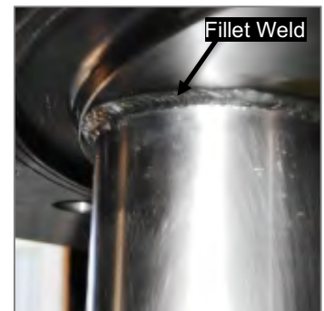
Figure 2-3 Fillet Weld
