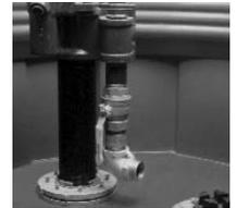
For swivel type piping connections, a plumbing assembly fitted with a standard plumbing elbow fitting would be connected to a swivel or barbed adapter. The arrangement accommodates the connection of a swivel pipe coupling installed on the end of a flexible pipe section.
