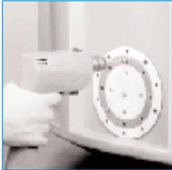
For proper installation, the appropriate size fabrication template should be used for accurate hole drilling.
