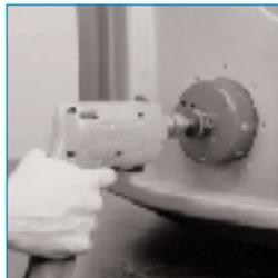
**WARNING: The appropriate hole saw size must always be used for proper installation of the flexible entry boot. Failure to use the required hole saw could damage the rubber boot after installation or prevent the boot from sealing properly and void product warranty.**
