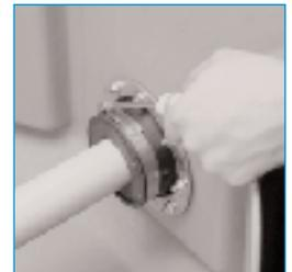
**WARNING: Do not over tighten the band clamp beyond the maximum torque of 30 inch pounds or it is possible to damage the rubber boot.**
