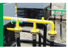
Manifold prepared to be fitted with safety relief valve.
