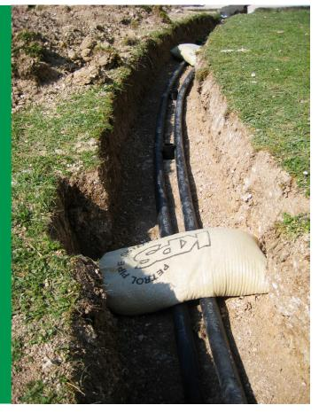
Use bags with sand to keep the pipes in place during installation.
