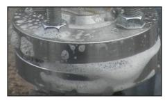
Perform tightness test with soaping before backfill.
