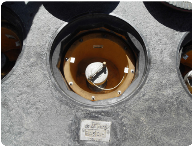
Fibrelite direct fill spill buckets (without drain back to tank) specified by Total
