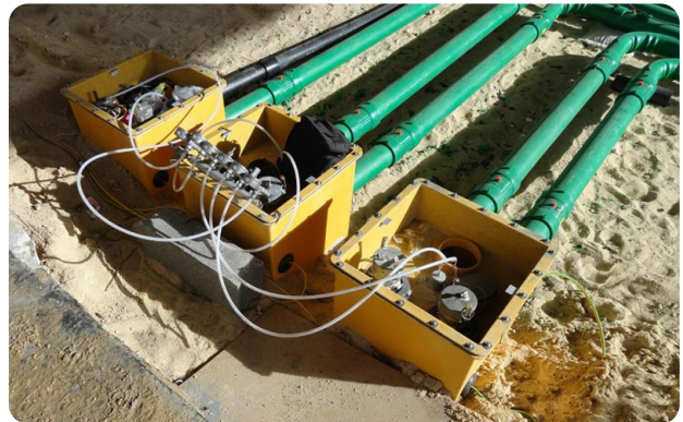
Secondarily contained Fibrelite remote fill sumps
