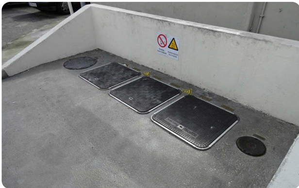
Recently upgraded site with Fibrelite's 600mm sq. 25 tonne load rated covers (FL60)
