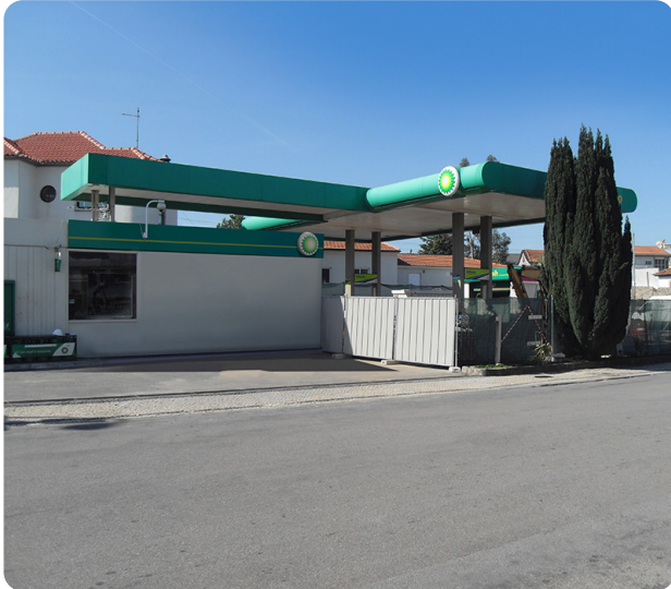
Site being upgraded with Fibrelite's fully conductive below ground remote fill sumps, covers and KPS conductive double wall fill pipe
