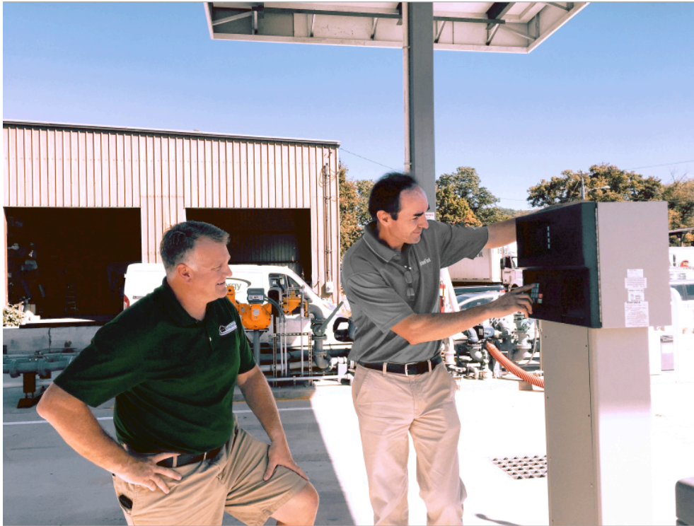
Simple Energy installed an integrated line of fuel management and loading equipment from OPW that eliminated the heating company's dependence on third-party fuel suppliers. The C/OPT™ Fuel Control System (shown here) provides 24-7 fueling authorization and accountability at Simple Energy's fleet fueling terminal in West Lebanon, NH.
