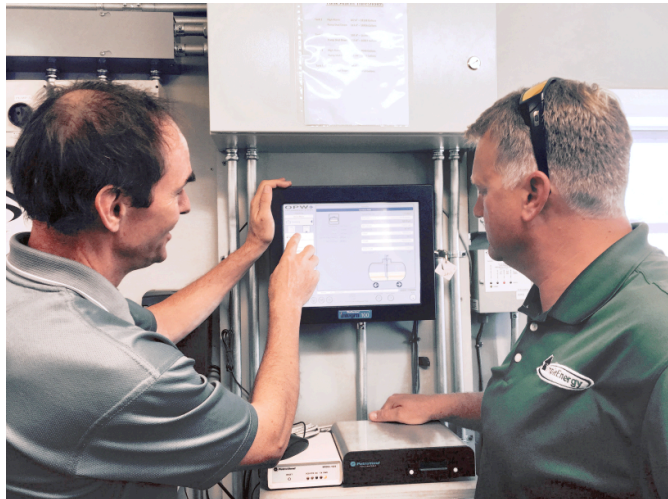
Simple Energy’s Rob Stenger (right) and John W. Kennedy Company’s Brian Devereaux (left) review inventory information on OPW’s SiteSentinel® Integra 500™ Console.
