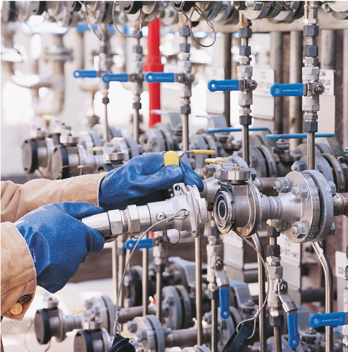
FIGURE 2. Numerous variables and components must be carefully considered when designing a loading system to ensure that leaks are kept to a minimum
