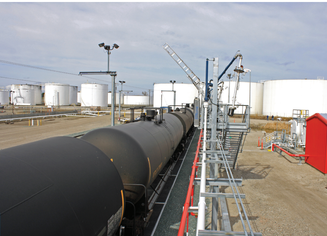
The Stockton terminal's new rail siding features six loading platforms
