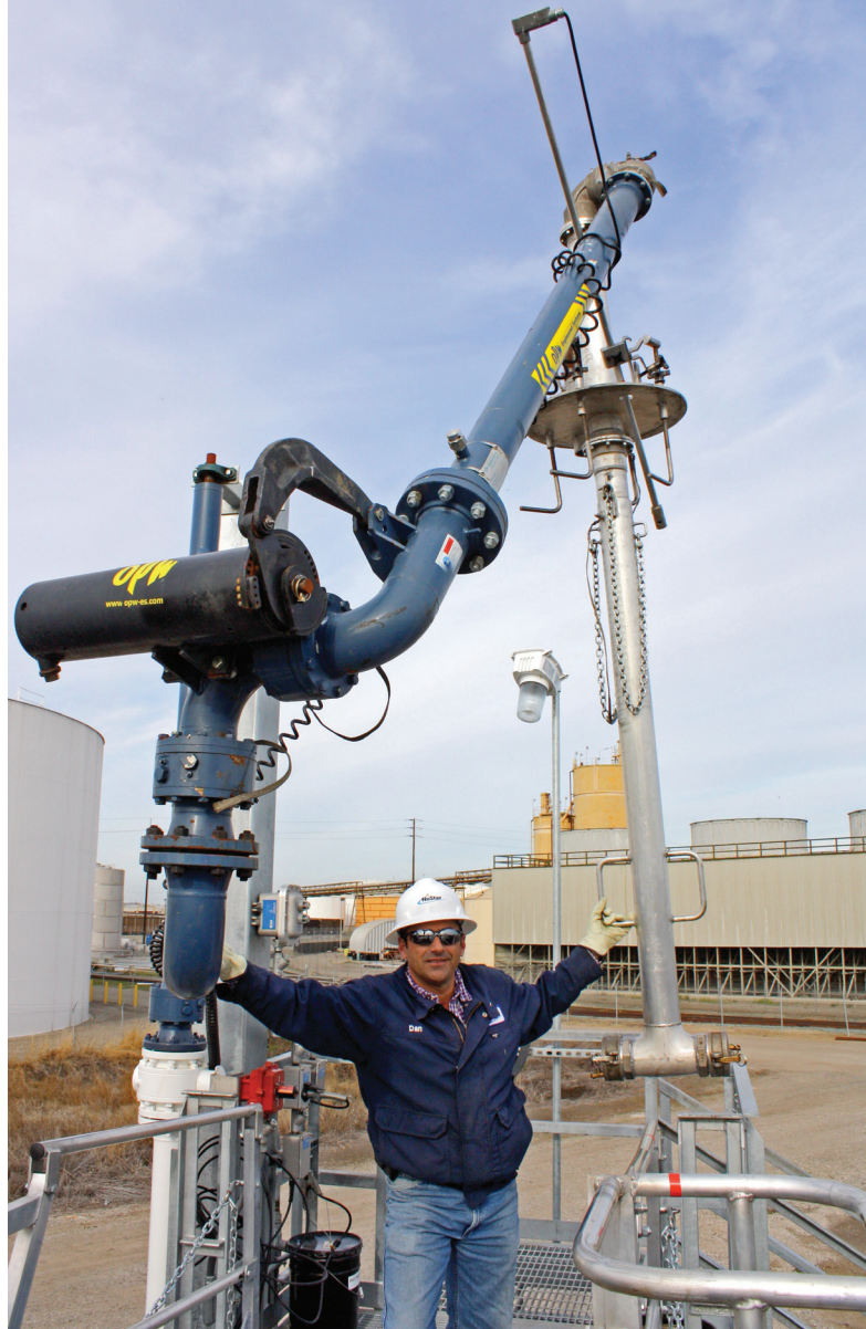
Dan Thomas, terminal manager at NuStar's Stockton facility, says he can't be more pleased with the new loading system
