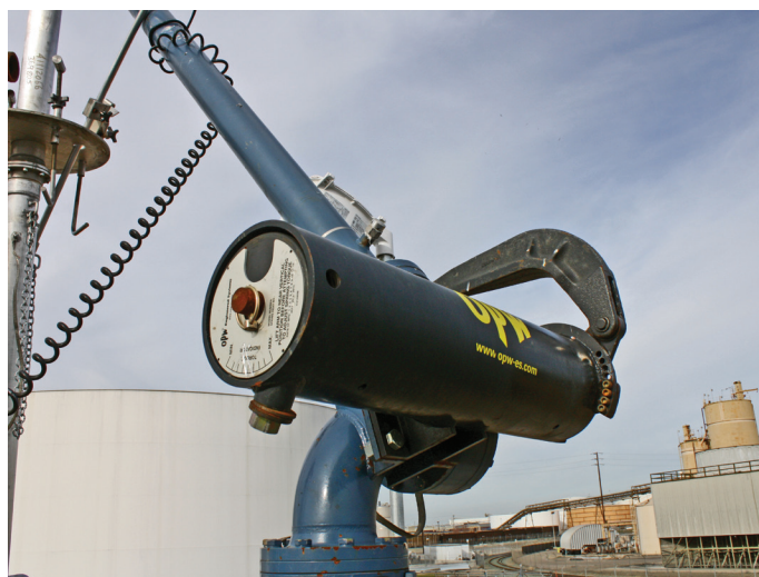
The 890 Series has been designed for loading arm systems that need to handle heavy loads and travel long distances
