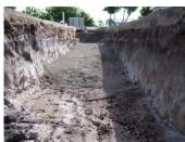
layer of bedding material under the pipe. Remove all sharp rocks and debris from the trench bottom before bedding material is installed.
