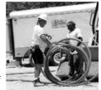
pipe as straight as possible for accurate measuring and marking for cutting purposes.
