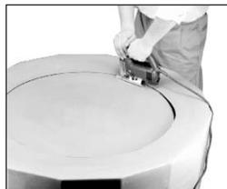
inside of the cut-out opening. Using two vice grips, clamp the ring to the sump base. Using an electric drill fitted with a 7/16" bit drill out the 24 bolt holes, remove the segmented ring from the sump base.
