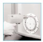
5/16" drill bit. After drilling, remove the template from the sump base wall.
