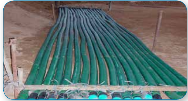
Straightening of coils.
