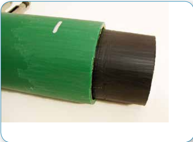
Correctly scraped pipes. Oxide has been removed from the whole area to be welded.
