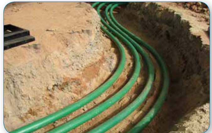
Coiled pipe laid in slight curves that allow the pipes to adjust to temperature changes or ground movement.
