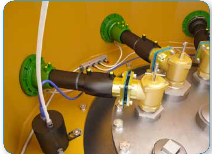
The KP 315 Leak Detection System.
