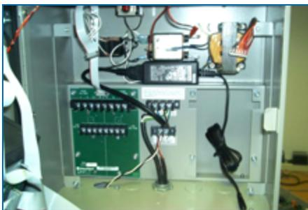
Figure 2-1 FIT-Mounted Modem Power Supply
