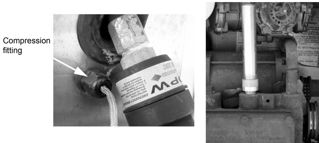
*Figure 6: Cable Compression Fitting and Intrinsic Barrier Installation*
